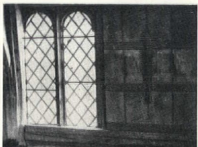
Sliding wooden shutter of the type originally used in unglazed openings. Sussex. Late C15
