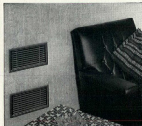
View in living room showing warm air outlet (below) and return air inlet.
