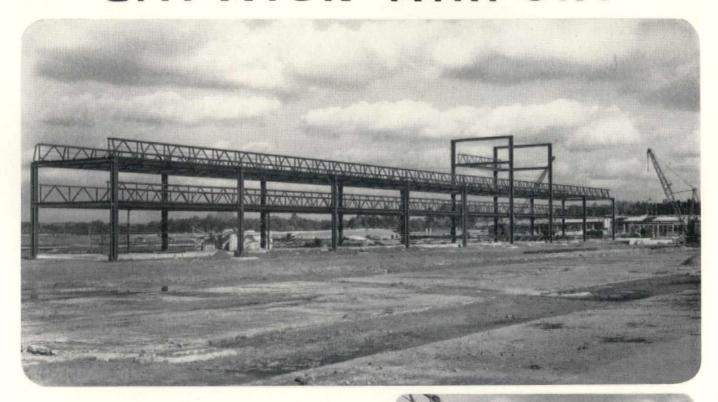
Hotchkiss Lattice Girders of welded tubular construction were supplied for the Central Pier. We are pleased to have contributed to this important development and are always enthusiastic to assist in the technical advancement of structural engineering.
