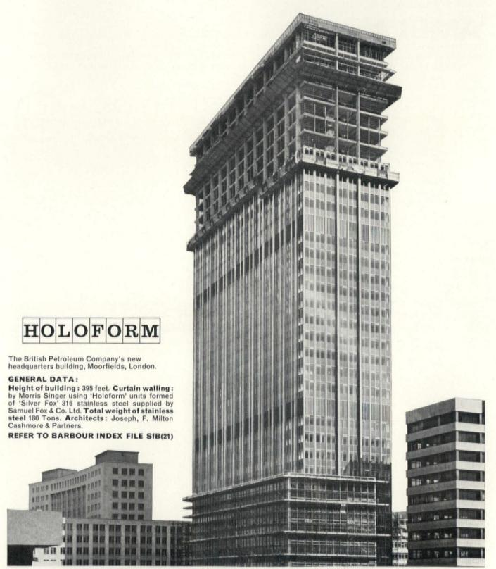
This impressive tower block, now nearing completion is totally enclosed with HOLOFORM curtain wall units formed of stainless steel. The long-term cost-saving advantages of simple
