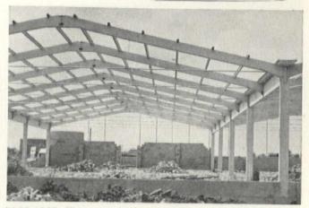
'I' FRAME: Tied arch, 111 pitch, precast reinforced concrete. Spans up to 60'. The 'I' frame is extendible by either additional spans or bays. 30' internal and external column spacings available.
