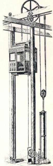
To display his confidence in his own safety device Elisha Otis at the Crystal Palace in 1853, cut the rope from which his lift was suspended, thus allaying the fears associated with passengercarrying lifts
