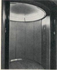
Circular, freestanding lifts in the Board of Trade Building, Victoria Street, London, by Otis Elevators Ltd., designed for high capacity and a particularly advantageous ratio of door opening width to the overall
