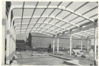
'F' & 'F2' FRAME: Low pitch portal, 1110 pitch, precast reinforced concrete. This series has now been extended to include the 'F2' frame offering a range of spans from 30' to 60'. These structures have been designed specifically for Industrial construction. 30' internal column spacings available.
