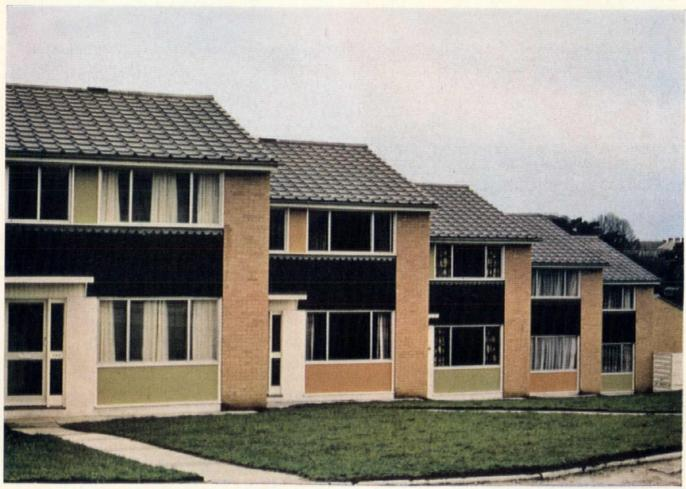
TURNALL COLOURPREST Asbestos-Cement Fully-Compressed Flat Sheets in use as Infill Panels below and between windows of each house on the Golden Valley Housing Estate, Sandgate, Nr. Folkestone, Kent.
