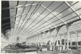
'A' FRAME: Portal frame, 22½° pitch, precast reinforced concrete, spans 15' to 60'. Standard bays 15', special bays to clients' requirements. An extremely versatile structure which may be extended in any direction, without prior provision, by the addition of further spans, bays or lean-tos.
