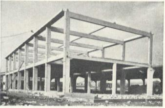
'K' FRAME: The 'K' frame has been specially designed for single- or two-storey flat roof office and industrial structures. It is based on a standard module and has a simplicity of construction permitting complete freedom of design and infilling with all conventional materials. Spans up to 36', bay lengths on 15' centres.
