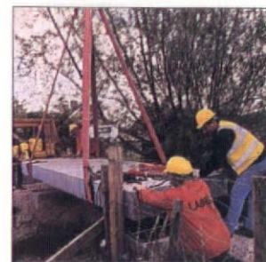
Chalgrove Bridge, the world's first concrete bridge with plastic reinforcement
