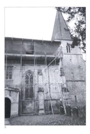
Dressed, 1995-96, Church of the Holy Rood, Sparsholt, Oxon, interventionary materials used on this Grade 2 listed building: oak, epoxy resin, mortar, steel, lead, lime mortar and others. Project undertaken by the author included replacement of existing lead roofs with new and extensive timber repairs for the client, the Parochial Church Council, Sparholt (fig 5)
