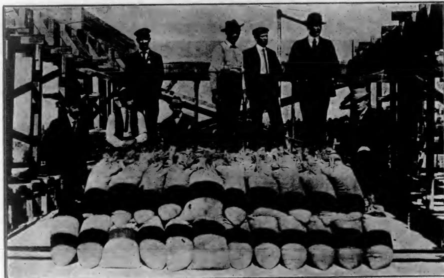
**T**ONS of sacks filled with sand were placed on the floors of the Bixby Hotel, causing a super-imposed load of 240 pounds per square foot. This load is six times the load for which these floors were designed, and is equivalent to the weight of three tiers of heavy men packed together as closely as possible, and one tier on top of another.
