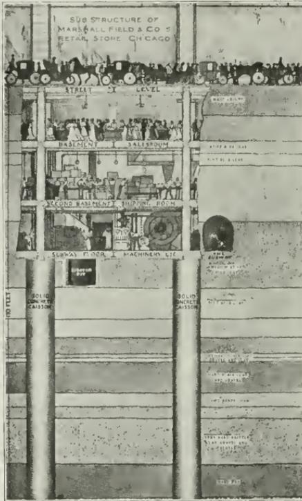
Sectional View Showing Foundation and Sub-Basements,
