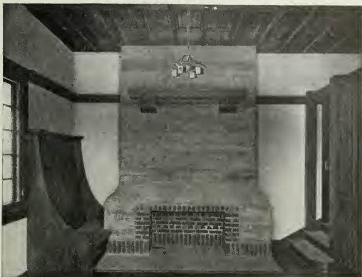
Fig. V.—Living Room Fireplace of Reinforced Concrete.
