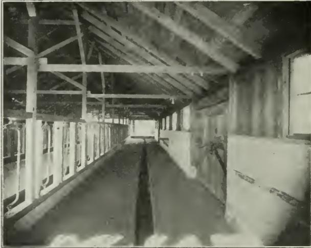
*Reinforced Concrete for Farm Buildings—Showing High Foundation Walls and Floor Drainage Arrangement*
