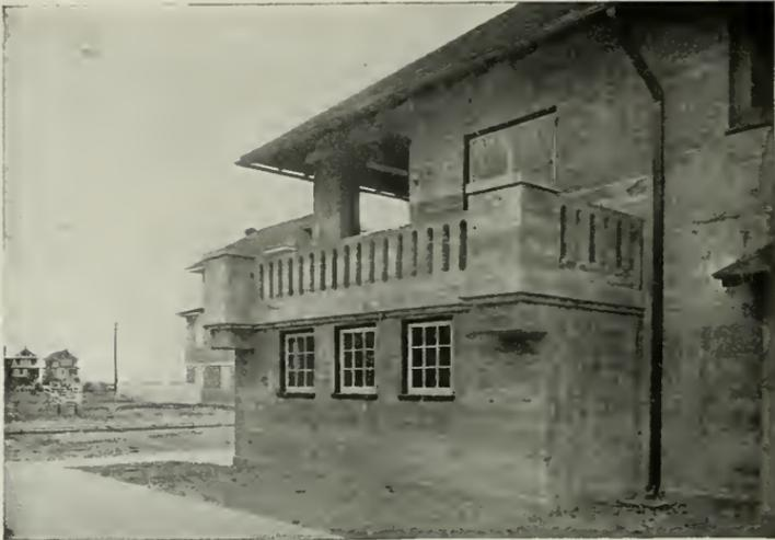
*Fig. I.—Detail View Showing Texture of Walls and Substantial Concrete Posts and Balustrade of Porch
