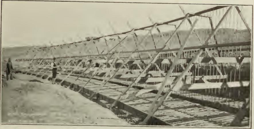
Showing Method of Reinforcement for Walls of Concrete Oil Tank near San Luis Obispo, California
