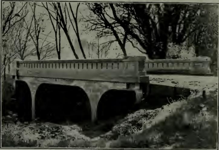
*A Reinforced Concrete Flat Slab Bridge, Ross, Marin County, California*
