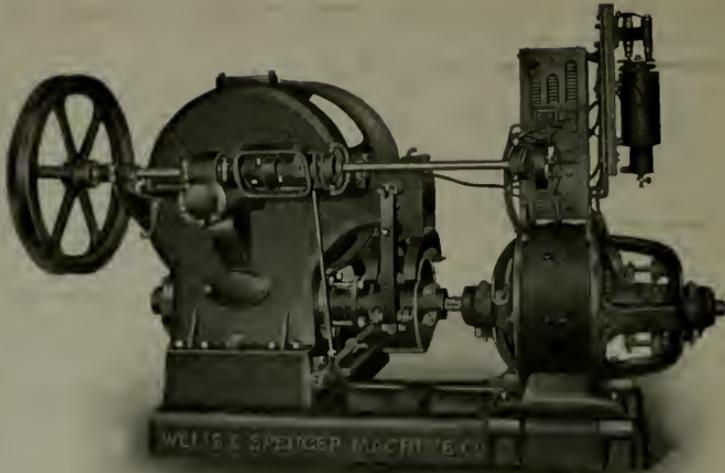
*This plate shows a Direct-Electric Freight Elevator Machine, the type being installed exclusively by the Spencer Elevator Company. The brake is cast in bloc with the gear casing, thereby making it rigid in every respect.*
