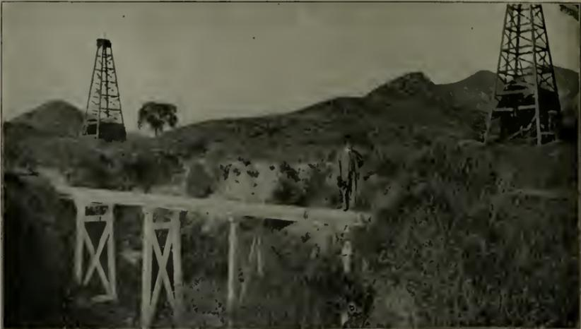
View of Corrugated Culvert Pipe Carried Over a Deep Arroyo on a Wooden Trestle Without Provision for Expansion and Contraction
