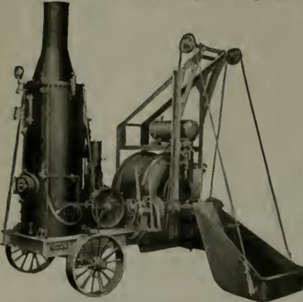
rollers keyed onto the shaft, preventing wobbly drums; its trucks with 100% safety factor of strength; and so on all throughout the entire machine.
