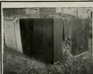
Manure test of Black Armco Iron, Plain Steel, and Copper-Bearing Steel. Armco Iron in good condition. Plain Steel badly corroded. Coppered Steel total failure
