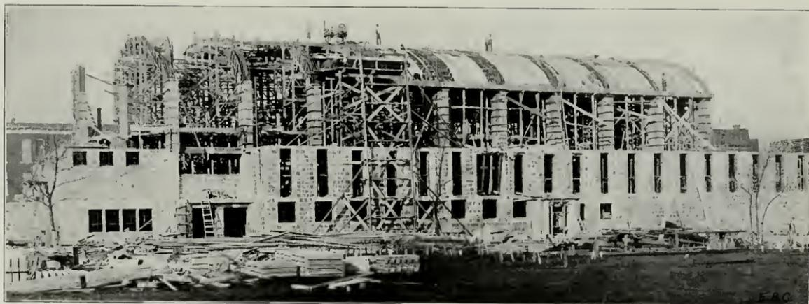
FIG. 6—EAST ELEVATION OF CHICAGO HEBREW INSTITUTE SHOWING ARCH AND ROOF-SLAB FORMS AND STAGING—VIEW ALSO SHOWS MATERIAL CARRIAGE HOIST
