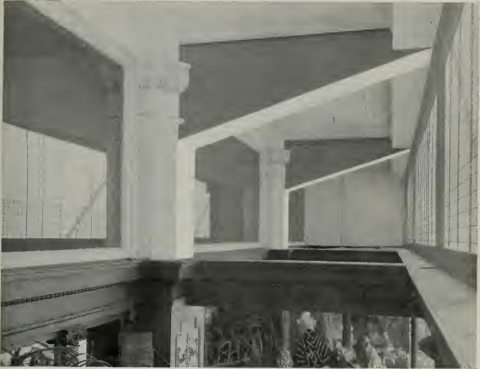
Fig. 11—SHOWING CANTILEVER CONSTRUCTION, HALE BROS.' DEPARTMENT STORE
