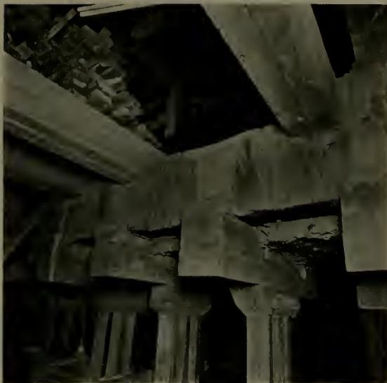
CONCRETED GIRDERS SUPPORTING OLD FOUNDATION. CONCRETE COLUMNS UNDER THEM BEARING ON SECTIONAL PILES
