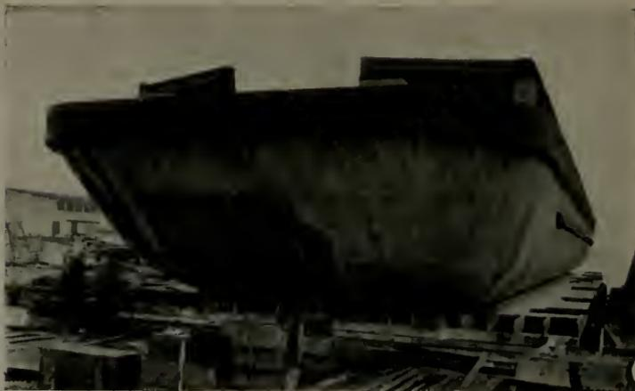
REINFORCED CONCRETE BARGE
