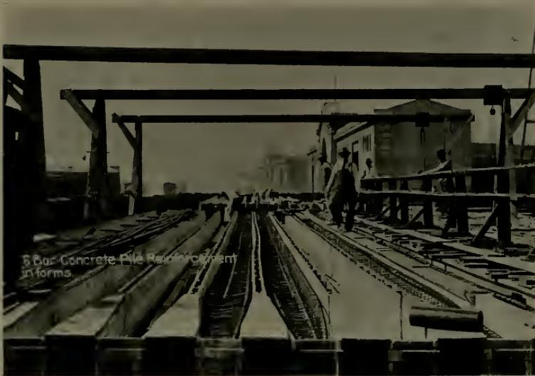
CONCRETE PILE REINFORCEMENT IN FORMS, PIER 31
