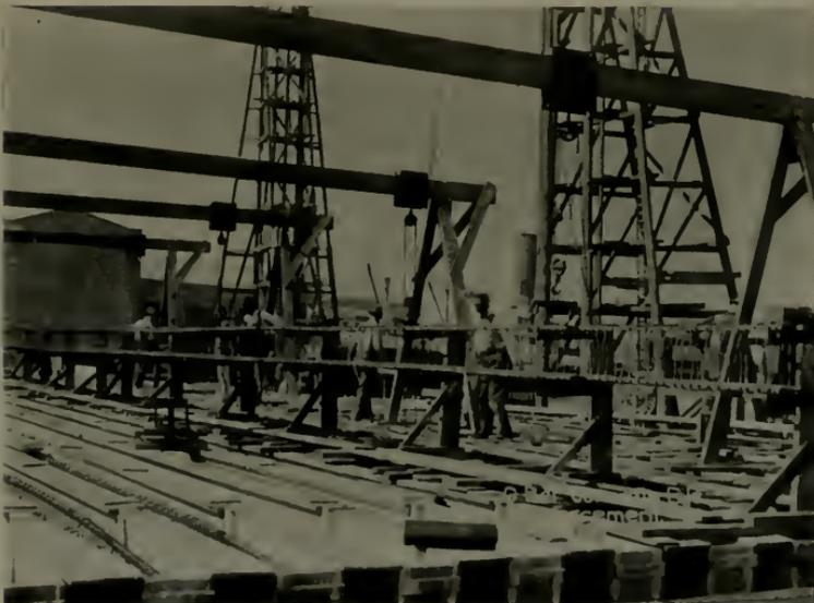
SIX BAR CONCRETE PILE REINFORCEMENT, PIER 30
