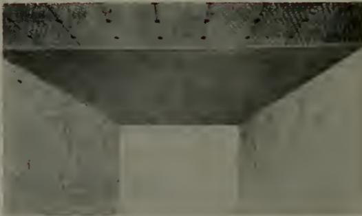
SUSPENDED CEILINGS GIVE UNIFORM PLASTERING SURFACE, are rapid in erection and perfect **BUTTONLATH** non-conductors of sound. They also have striking advantage of low cost combined with severely tested capacity for fire resistance.
