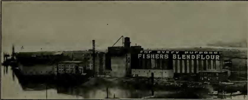
Fisher Flooring Mill, Seattle, Wash. 125 tons of black and galvanized Armco Iron used for roofing, ventilators, bins, hoppers and chutes.
