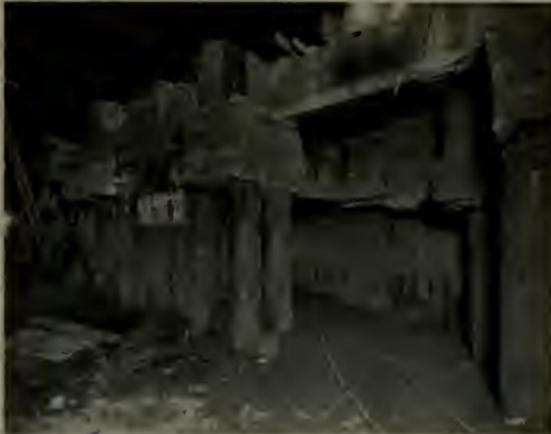
UNDERPINNING PILES SUPPORTING CONCRETED GIRDERS WITH SUBWAY ROOF BEAMS ON TOP
