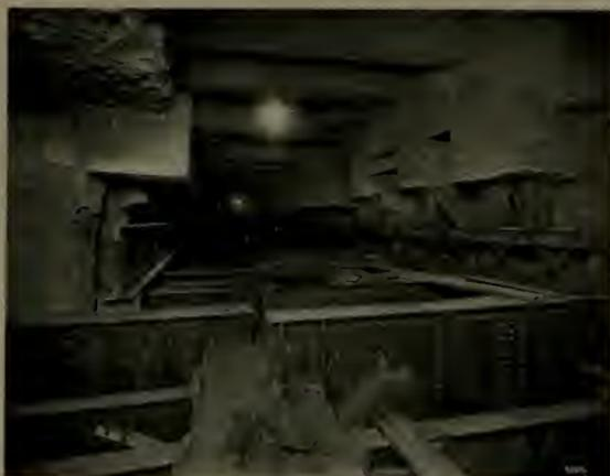
LATTICE GIRDERS INSTALLED ON SUBWAY ROOF BEAMS
