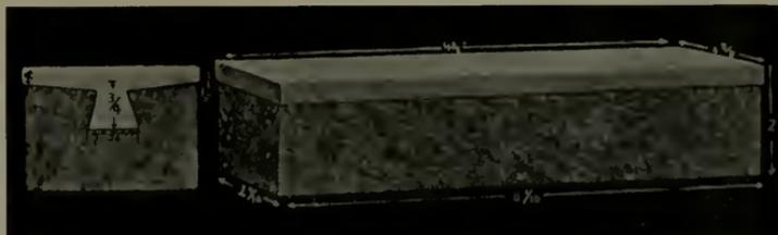
**GLASS BRICK** has been found to possess both artistic and structural merits. Manufactured in any desired tone—bright or subdued—a substitute for Clay Brick for Exterior Walls of Hotels, Apartment Houses and Hospitals.
