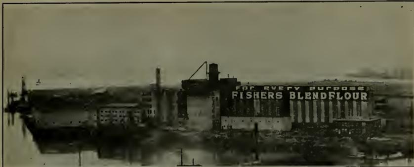
Fisher Flouring Mill, Seattle, Wash. 125 tons of black and galvanized Armeo Iron used for roofing, ventilators, bins, hoppers and chutes.
