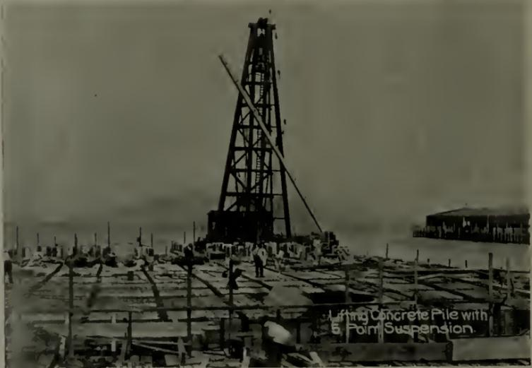
LIFTING CONCRETE PILE WITH FIVE-POINT SUSPENSION, PIER 3,
