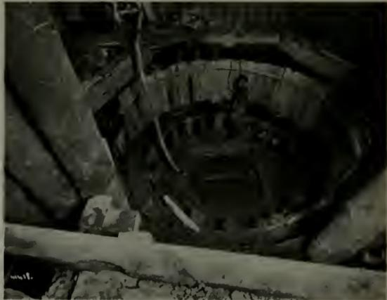
SUMP PIT EXCAVATED AND SHEET PILED WITH CONCRETE WALL FORM PARTLY ASSEMBLED
