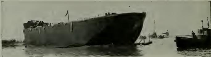
The Concrete Ship "Faith." Length, 336 feet. Beam, 44 feet. Capacity 5,000 tons.
