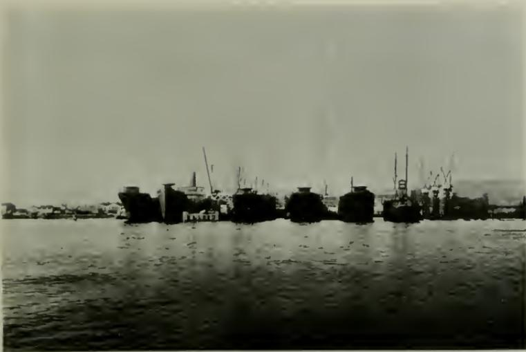
HULLS AT FITTING-UP BERTHS, AWAITING MACHINERY
