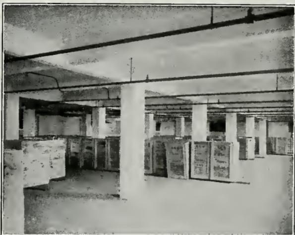
INTERIOR OF A STOREHOUSE AFTER FIRE. NOTE CONDITION OF THE CONTENTS AND THE SPRINKLER HEAD THAT WAS NOT FUSED INDICATING LOW TEMPERATURE AT ALL TIMES.
