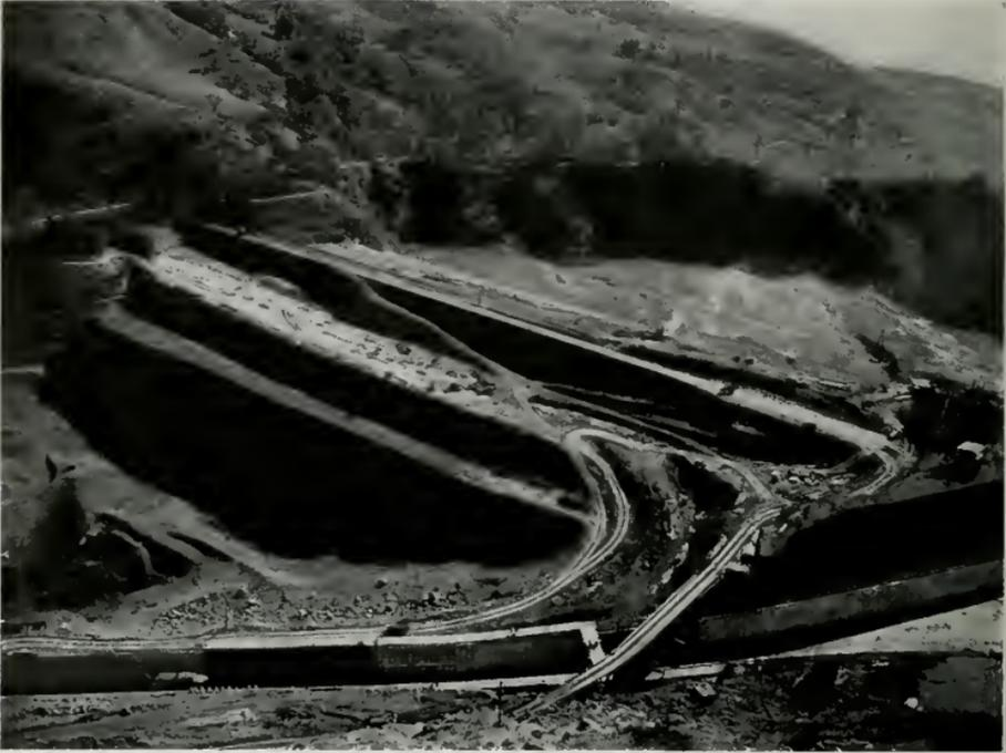
CALAVERAS DAM CARRIED TO A HEIGHT OF 215 FEET ABOVE ITS FOUNDATION, SHOWING BERM CONSTRUCTION OF THE DOWN-STREAM SLOPE
