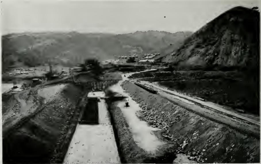
ROLLED CLAY CORE OF CALAVERAS DAM UNDER CONSTRUCTION. THIS CORE IS SUPPORTED BY THE EMBANKMENTS OF ROCKY MATERIAL
