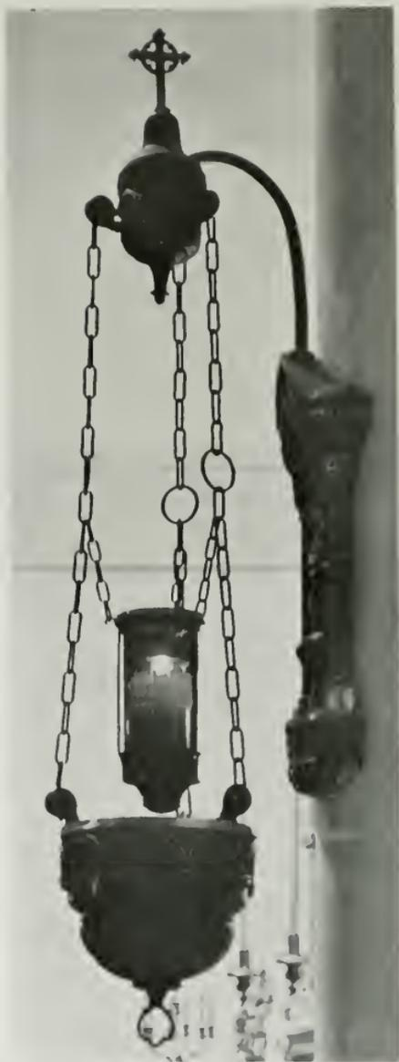
The main fixtures, suspended from 70 foot arches, are fourteen feet six inches high, carry thirty-two candles and weigh 1350 pounds each. The fixtures may be lowered by means of a windlass.
