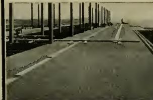
STEELEX Floor Lath is unrolled over the joists. The illustration above shows STEELEX Floor Lath in an unbroken stretch of 212'.
