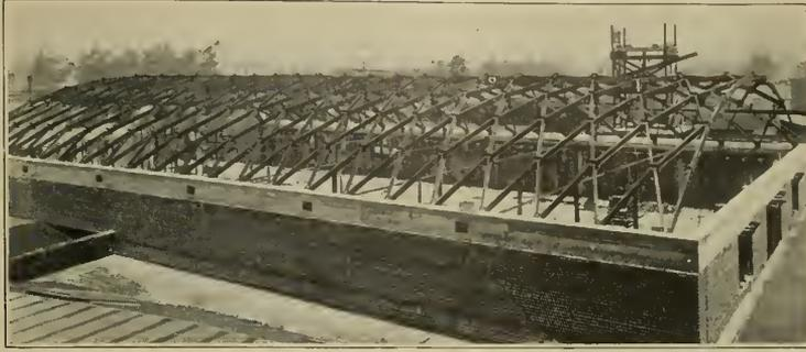
STEEL LAMELLA ROOF, COCO COLA PLANT, LOS ANGELES. THIS ROOF HAS A 70-FOOT SPAN
