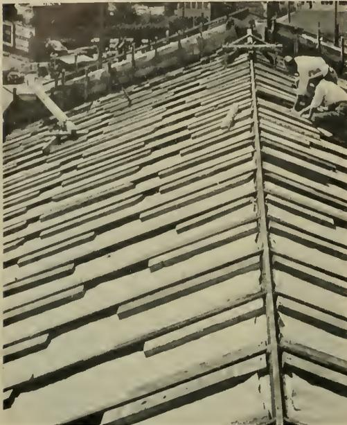
THE application of Sisalkraft for curing and protecting floors, ramps, stairs and sidewalks is common. Its use on pitched roof slabs as illustrated is a little unusual but none the less practical. Sisalkraft is laid in 22 inch strips between form dividers.
