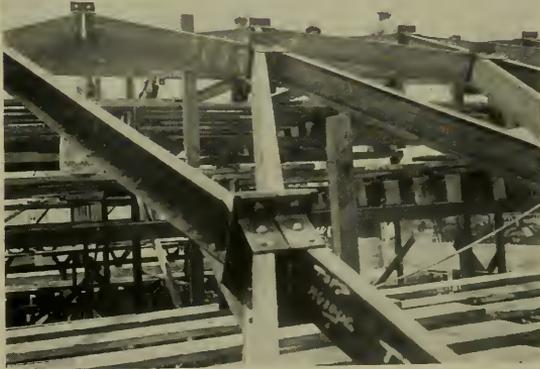
BRACKETS RIVETED TO ENDS OF STEEL CHANNEL LAMELLAS AND
