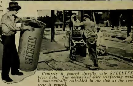
Concrete is poured directly onto STEELEX Floor Lath. The galvanized steel reinforcing mesh is automatically embedded in the slab as the concrete is poured.
