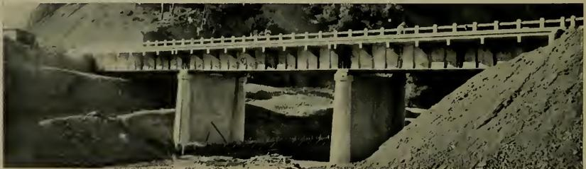
View of bridge after taking the surgical treatment that dismembered it and turned the 80-foot steel girders bottom-side up. It is now a perfectly modern structure with a 34-foot roadway, spanning Los Alamos Creek, on the new Ridge Route alternate.
