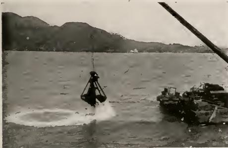
CLAM SHELL BUCKET USED TO REMOVE ROCK BLASTED 100 FEET BENEATH THE WATER
