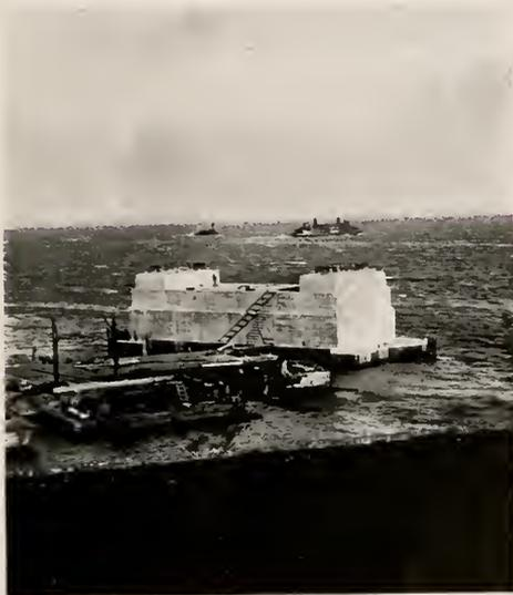
The first pier completed for the San Francisco-Oakland Bay Bridge, foot of Harrison Street, San Francisco. The pier stands 40 feet out of water and is 52 feet wide by 122 feet long.
