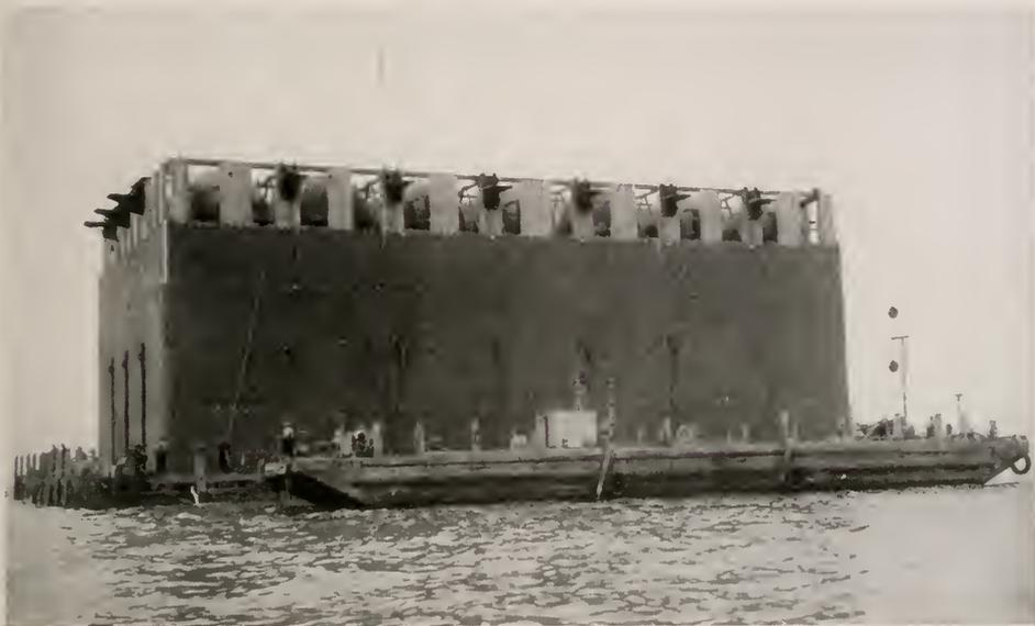
WEST BAY CAISSON A steel and timber structure the size of a small apartment house, anchored 1100 feet west of Verba Buena Island where it will be sunk to rock approximately 170 feet below the water line to establish the most easterly tower of the suspension sector of the San Francisco-Oakland Bay Bridge. This caisson is 74 feet wide, 127 feet long, 65 feet high, drawing 20 feet of water, and contains 28 steel cylinders, each 15 feet in diameter, now filled with compressed air to supply buoyancy.
