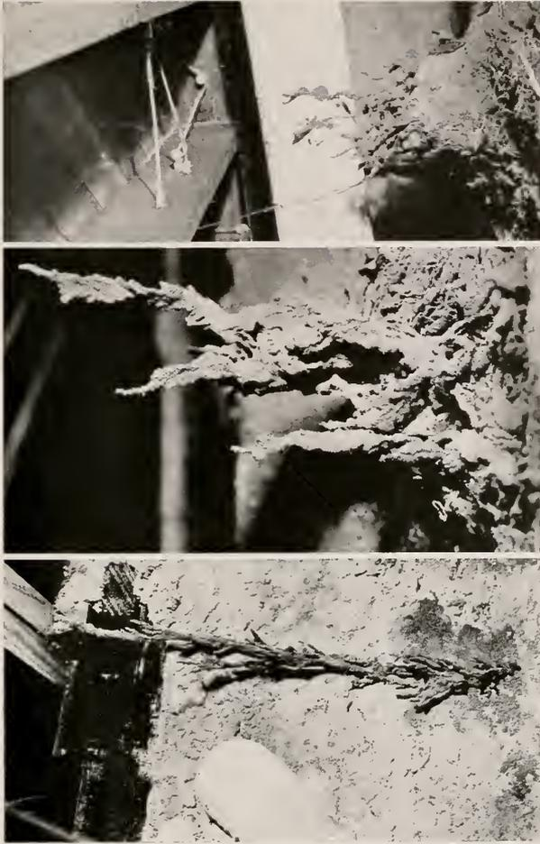
Fig. 5—Runways, tubes and towers made by subterranean termites under houses. Top—Branched tubes originating from a wood spreader embedded in concrete foundation. Wood forms had been left on the outside concrete wall of the building, which was only two and a half years old. Center—Towers of the western subterranean termite. Bottom—Towers and tubes of the western subterranean termite, from a stump left under a house.
