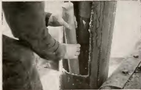
PICTURE SHOWS METHOD OF PLACING PILOT BOMB IN CHUCK AT END OF STEEL SPUD
