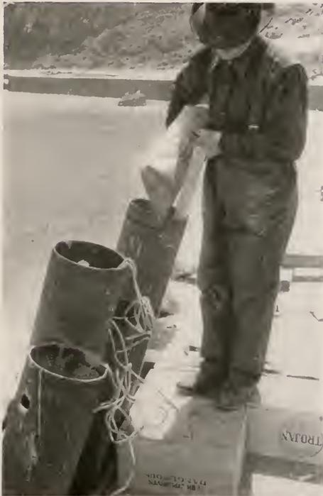
LOADING large casing bombs with 60 per cent dynamite. The bombs are 8" in diameter and 22' long. They hold from 100 to 350 pounds of dynamite.
