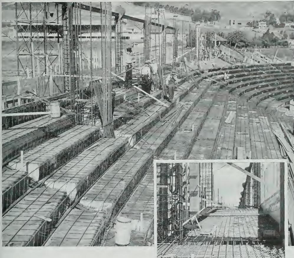
THE Live Stock Exposition Building, now under construction at Visitacion Valley, is but one of many structures on the Coast in which Bethlehem Reinforcing Bars are used. Others are the Bonneville Dam, the anchor blocks of the Golden Gate Bridge and conduits of the Metropolitan Water District Aqueduct.
