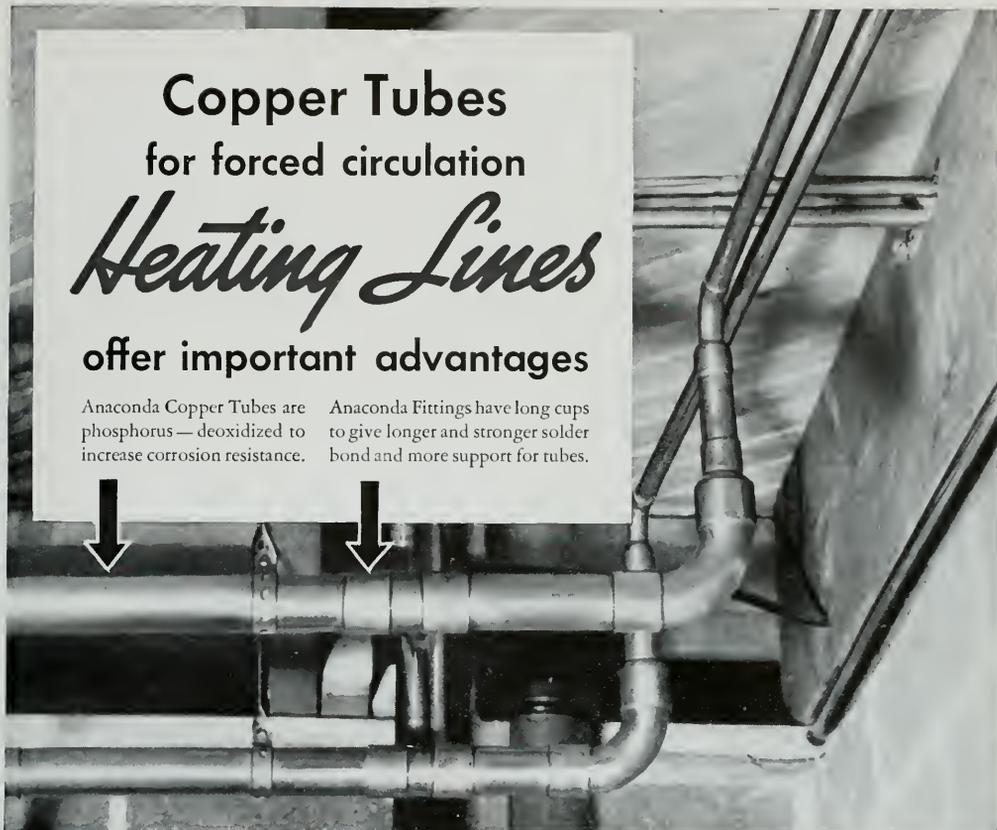
HERE'S the best value in piping, not only for hot and cold water and air conditioning lines, but for the heating system as well. For heating lines, Anaconda Copper Tubes mean a lower heat loss. On most jobs, insulation is unnecessary. And smaller sizes can almost always be used because the smoother inside walls of copper tubes permit a higher rate of water flow. More heat is delivered—faster! Yet these non-rust tubes cost little
