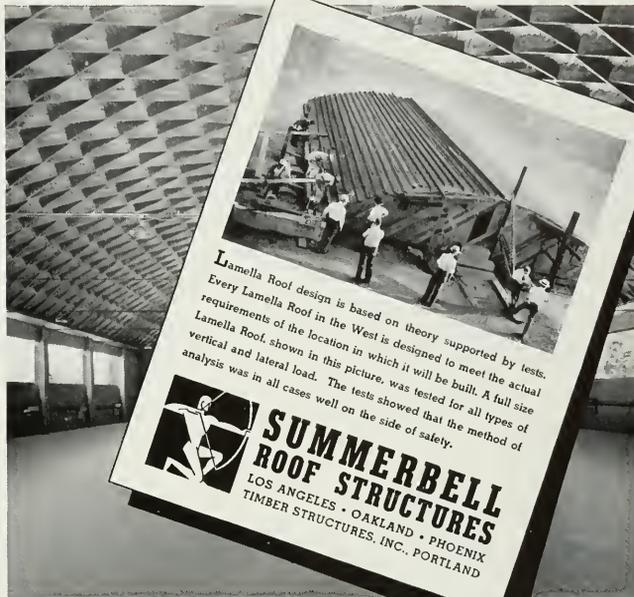
Lamella Roof design is based on theory supported by tests. Every Lamella Roof in the West is designed to meet the actual requirements of the location in which it will be built. A full size Lamella Roof, shown in this picture, was tested for all types of vertical and lateral load. The tests showed that the method of analysis was in all cases well on the side of safety.
