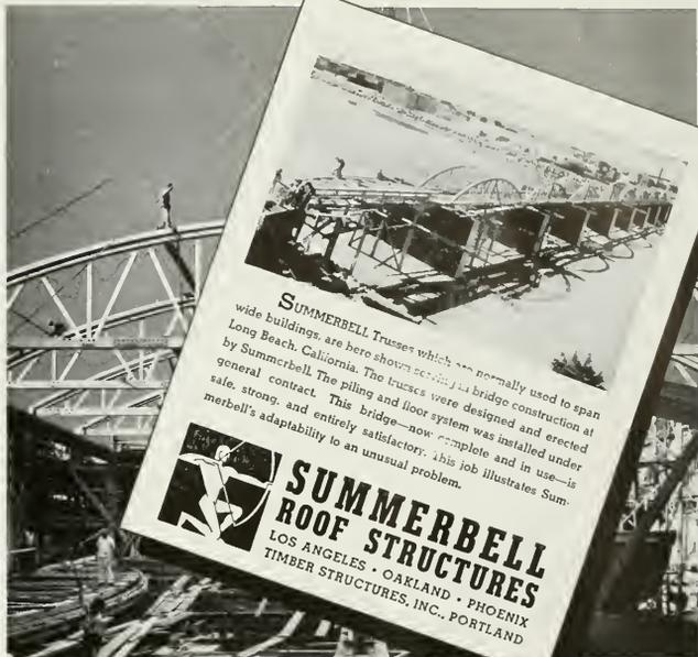
SUMMERBELL Trusses which are normally used to span wide buildings, are here shown spanning a bridge construction at Long Beach, California. The trusses were designed and erected by Summerbell. The piling and floor system was installed under general contract. This bridge—now complete and in use—is safe, strong, and entirely satisfactory. This job illustrates Summerbell's adaptability to an unusual problem.
