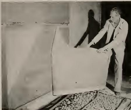
from the concrete, after the forms have been removed, leaving a surface which is smooth and attractive in appearance without refinishing.
