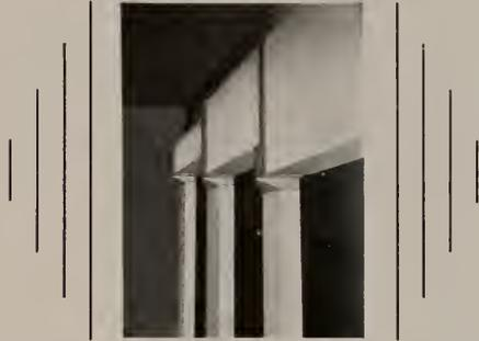
The duct is acceptable in residential installations carrying normal temperatures in either gravity or blower types and can be used up to within six feet of the plenum chamber on the supply line and the entire return line.
