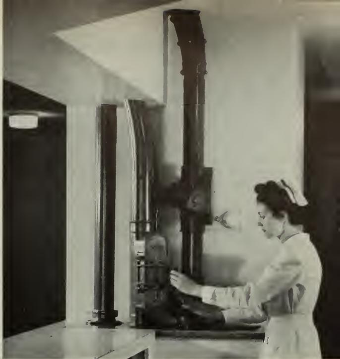
**Tube Stations such as this one enable the tubes to do double duty since carriers can be sent to the Central Tube Desk from more than one point on the same line.**
