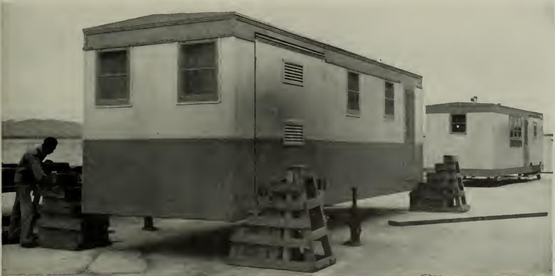
**Simple method of loading and unloading a Wingfoot Home with little equipment calls for the use of jacks and house steps. The house is jacked up gradually to a height sufficient to back a trailer beneath it. Note that bedroom bays are collapsed to permit movement on the highway.**
