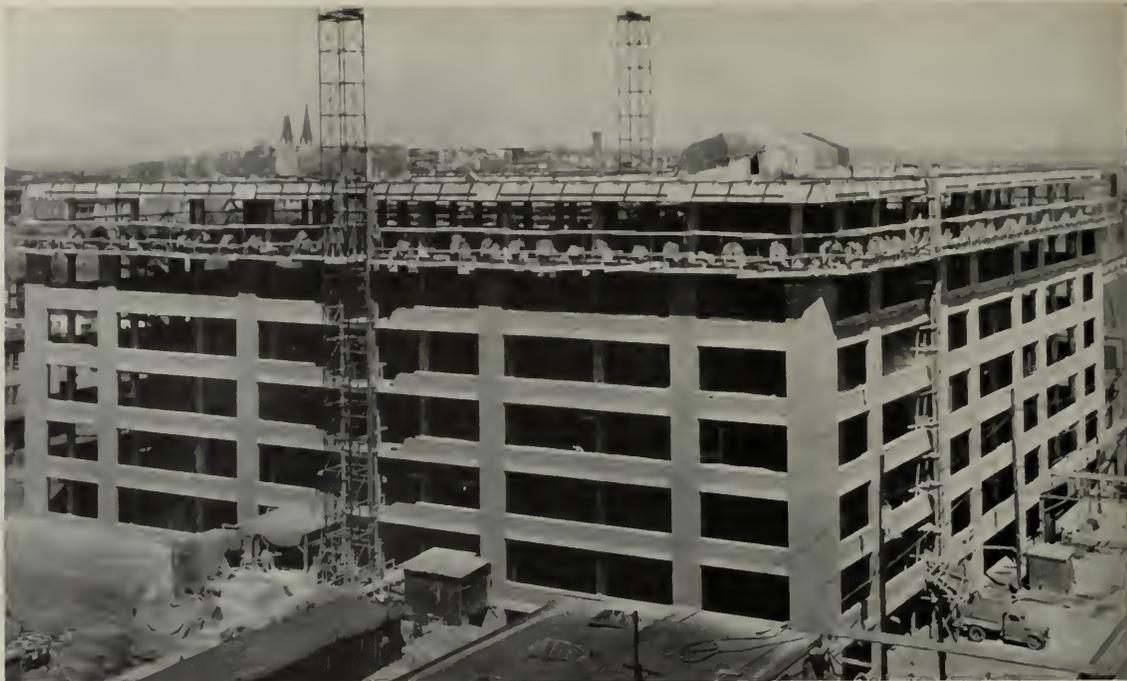
**UPPER VIEW** is the new six and one-half story building of reinforced concrete and brick construction with an area of 240,000 square feet which is being built by **THE STANLEY WORKS, INC.**, of New Britain, Conn. It will house machinery for manufacture of regular hardware lines on an expanded scale to meet postwar requirements of the firm.
