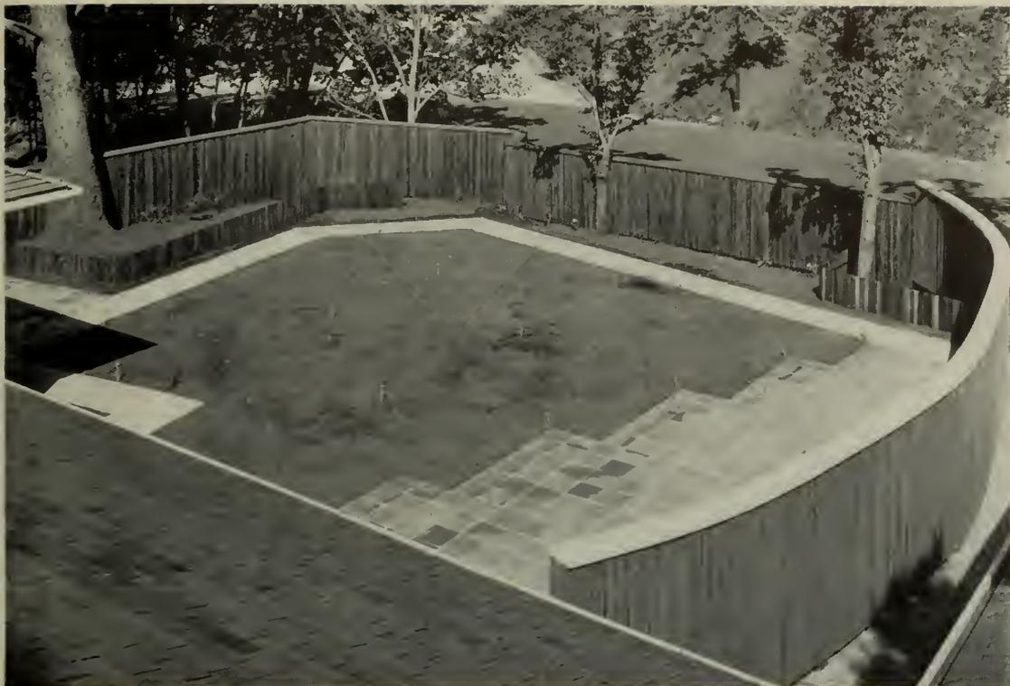
**THE ABOVE** illustration shows the court in its present state of completion; the lower forward wall is redwood bark with a finished redwood cap painted similar to the house exterior. Paving and planting intergration. This forward court, which utilizes space normally left open to the public, solves the problem of entrance access and privacy thus permitting maximum land use to the owner.
