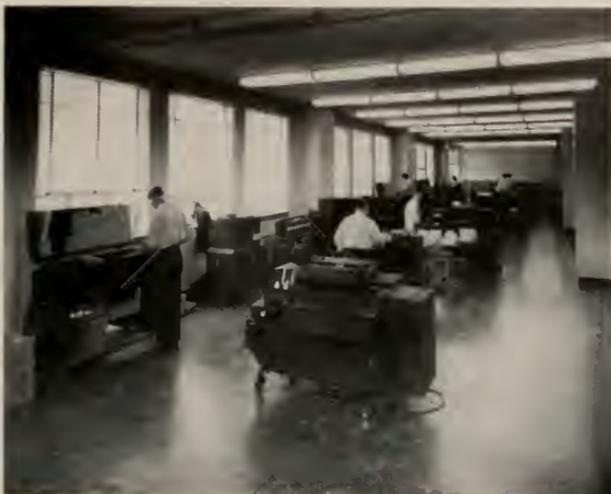
Lighting is provided by cold cathode lighting which is supplemental to a great deal of natural lighting. Floors are of asphalt tile and movable steel partitions permit an expansion or consolidation of any department without having to do a major remodeling.
