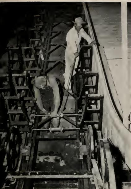
The vertical brackets alongside the electric stairway tracks support the balustrade on which the handrail travels. Both stairways are reversible; they can be set for up-going traffic on right with down traffic on left (See photographs on Page 29).
