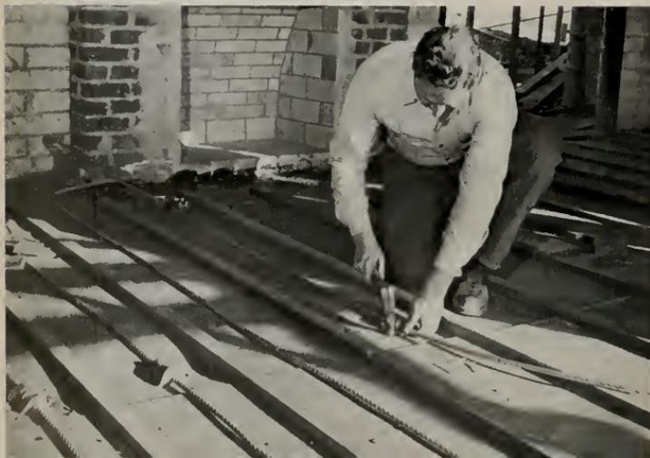
Wire Rope Cables are laid over glass wool floor insulation with special clips for floor.
