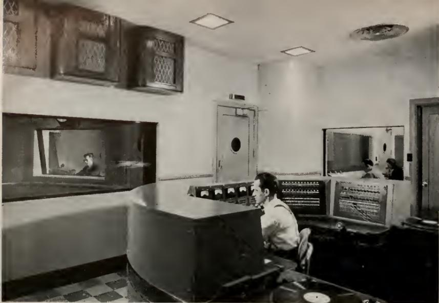
**CONTROL ROOM.** The ingenious arrangement of control facilities has drawn notional attention to KOMO. From his seat at the master control console, this engineer can see into the two 2-way control booths which serve three smaller studios located side by side on the left. He also has visual contact with the operations control center through the window on the right, and with the recording department which also adjoins the master control room.
