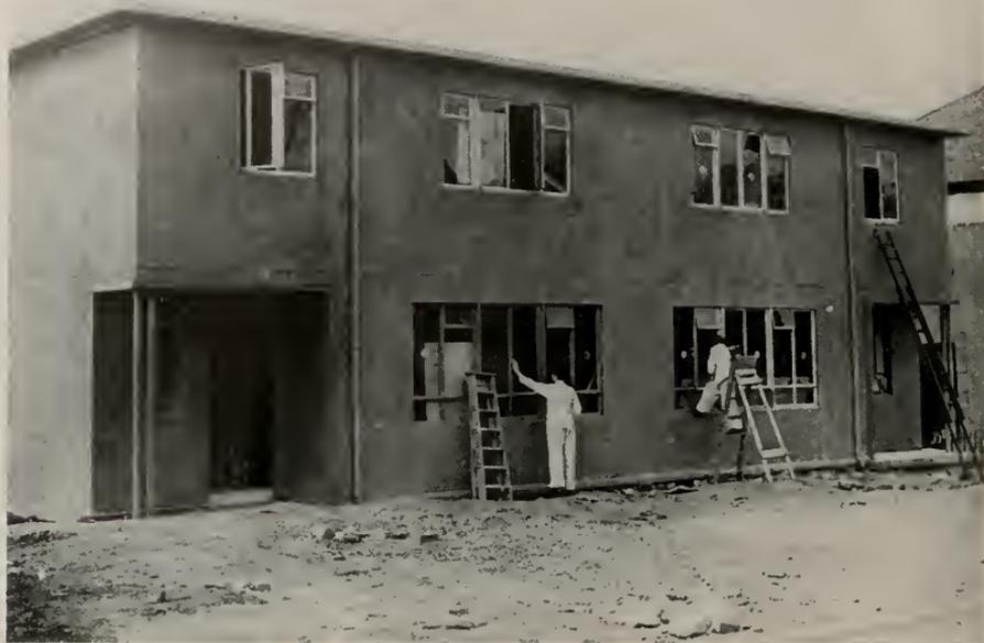
**FIRST WEIR STEEL PREFAB SEMI-VILLA. Painters line off window frames and put the finishing touches to the first Weir steel house in Knightswood, Glasgow.**
