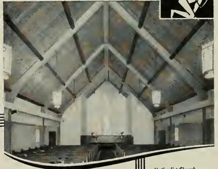
SUMMERBELL glued laminated arches and beams give the Architect the widest latitude in designing for the modern or the traditional...for the large cathedral or the small chapel. In addition to their lasting beauty, they provide structural advantages which effect substantial economies in overall costs. Write for illustrated brochure.
