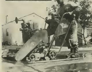
Some 1800 ft. of 9" Macadam base asphalt roadway was cut to a depth of 3 3/4", in accordance with specifications of the city, in a matter of 12 1/2 hours, or an average of 2 1/2 ft. per minute.
