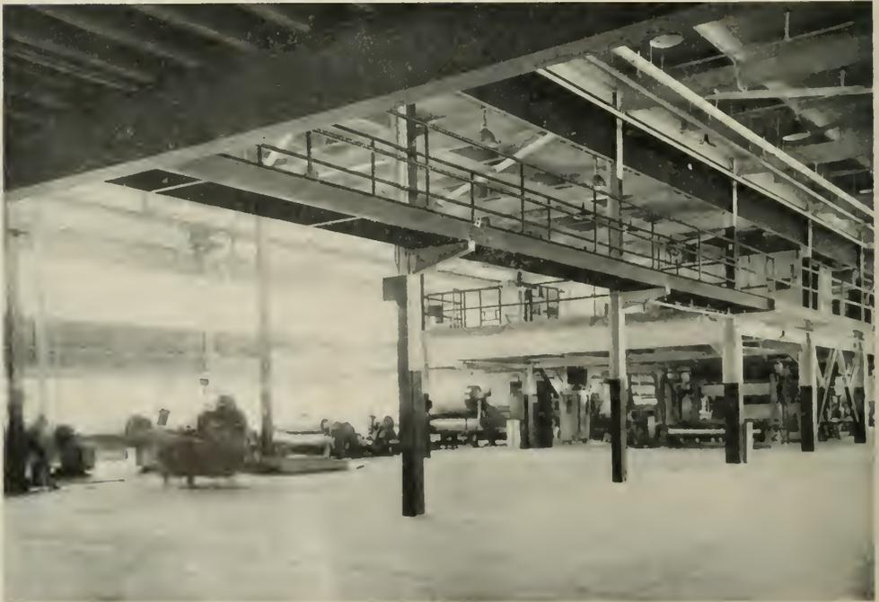
Glare and heat reducing glass, blue in color, is set in the steel sash. Cool-shade screens cut out south sun in mezzanine office and locker room areas.
