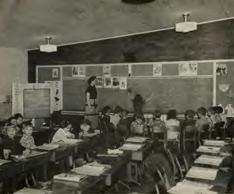
Economy roof rafters become ceiling joists for classrooms. Note pitch of roof against far wall. Acoustical tile ceilings give good results here . . . blackboards placed against end brick wall.
