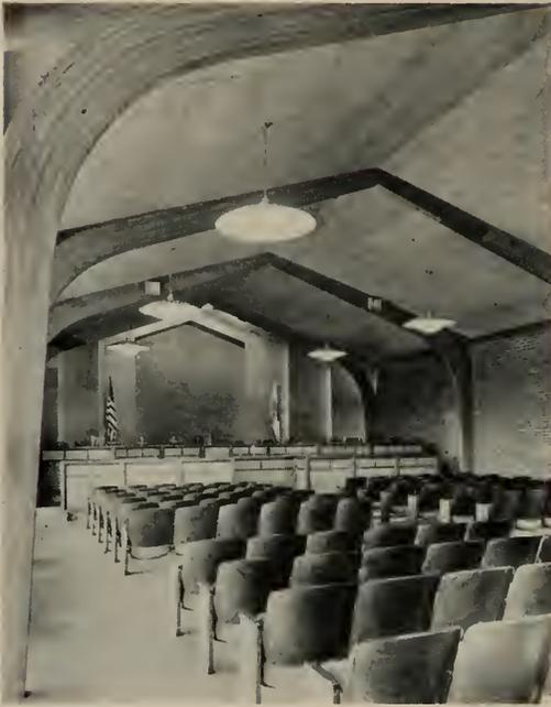
designed the Compton-Imperial Housing Project Auditorium. He says: "Wood laminated trusses were used on the project to meet the general design problem of clear span requirements as well as pleasing form. In addition, the wood trusses offered the necessary fire-rating and a more economical solution."
