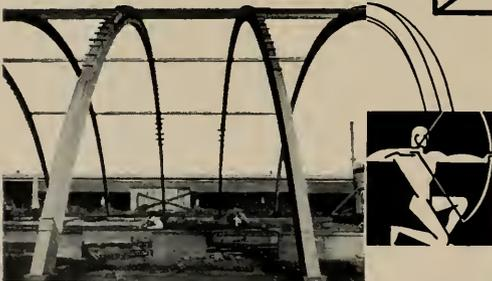
SUMMERBELL glued laminated arches, in any curvature and span desired, make it easy to plan gymnasiums and field houses totally free of obstructions. Fire safety, ease of erection, flexibility for all types of lighting and provision for large door and window openings are a few of the additional advantages. Write for illustrated brochure.
