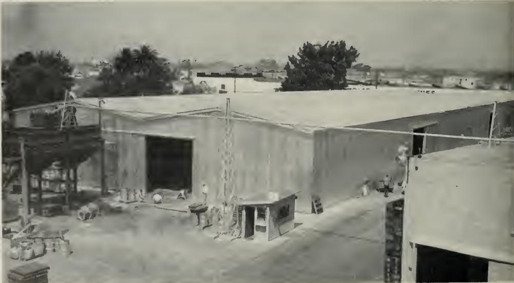
No technical difficulties of an unusual nature have yet been encountered. Basically, the structure resolves itself into a pressure-treated pole sunk in the ground. Vertical forces are carried by end bearing and skin friction, lateral forces by cantilever action of the pole.
