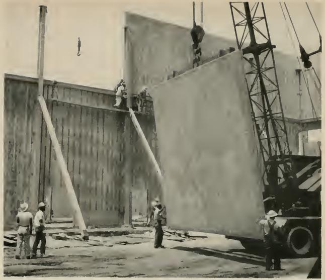
Using up to the minute construction techniques some eighty-four precast concrete wall panels were prepared and installed in a recent four days.
