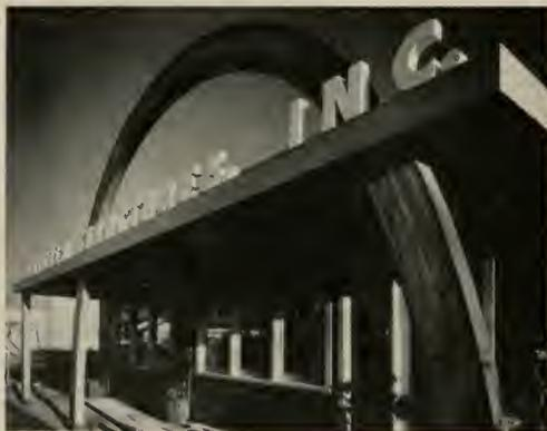
Glued-laminated arches of our own design and manufacture provide functional as well as distinctive framing for our own office building, subject of this month's cover of Architect & Engineer, John J. Moore Company, Engineers and Builders.
