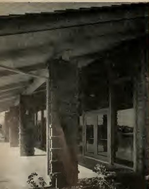
Purlins cantilevered beyond their supports in such manner as to reduce the interior moments and reduce the structural cost at the same time, providing the attractive shelter. Also shows how unusual surface textures may be introduced into grouted reinforced masonry.
