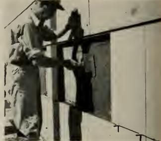
**3** To insure permanent bond between Veneer and structure, the wall surface is also brush-coated with the same Portland cement mixture.
