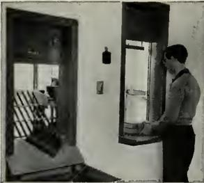
The conveyor consists of a vertically moving chain bearing finger type carriers; adjusted to unload at each receiving station and marked accordingly by a number of distinctive color. May be arranged for loading or unloading at any number of floors. Loading is done manually directly into the carriers on the "up" side of the carriers, unloading is completely automatic on the "down" side.
