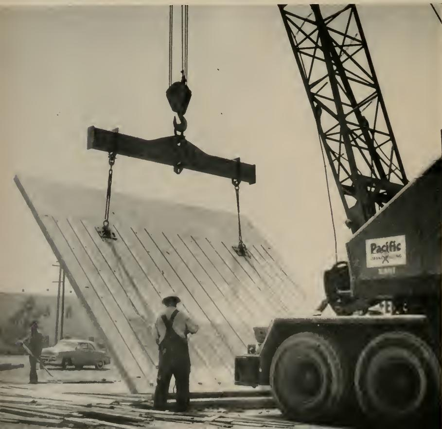
Shown here are the two tiers of 20 ft. wide precast concrete wall panels that make up the 46 foot high walls.
