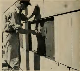
**3** To insure permanent bond between Veneer and structure, the wall surface is also brushed with the same Portland cement mixture.
