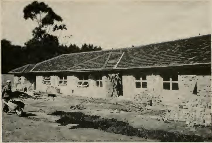
**THE CELLS—8'9" by 12'6" and 8'9" by 5", are transported to site and bedded down on standard foundations. Standard brick veneer and marseilles tiles gave this row of units the appearance of a much more expensive construction.**
