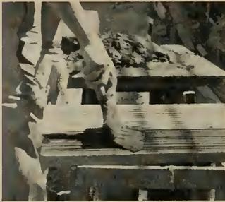
**2** Immediately before setting, the back of the Ceramic Veneer unit should receive a brush coat of neat Portland cement and water.
