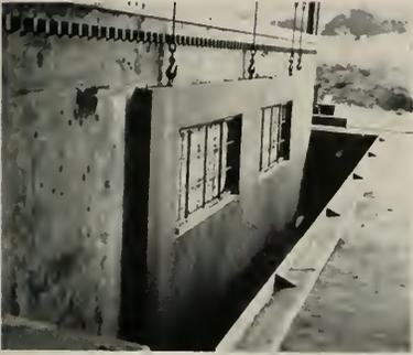
**WALL PANEL** ready for stripping. Table "tilts" to vertical positions to allow panel to be handled in this position until installed in walls.
