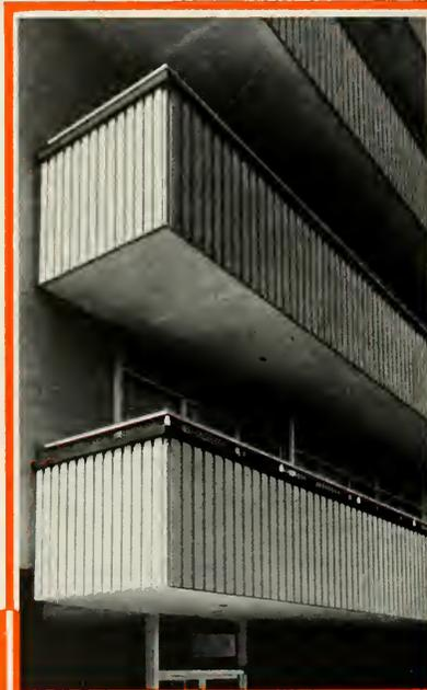
CONTRA COSTA COUNTY ADMINISTRATION BUILDING. Architectural Porcelain used to face building above first floor...for canopy facia...balcony and parapet caps... water table...and corrugated panels on penthouse and balconies.
