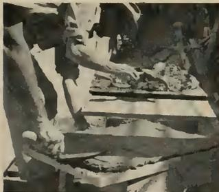
**4** Next, slightly more than  $\frac{3}{8}$  of an inch of mortar is applied to the C.V. unit. The same amount is also applied to the wall area.
