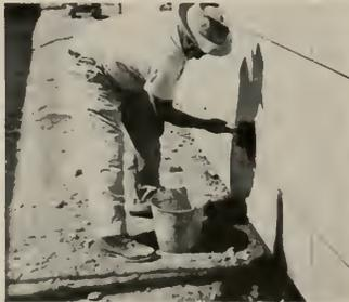
**8** Face joints may be raked out and pointed with fine mortar. To complete the job, surface is washed with clean water.
