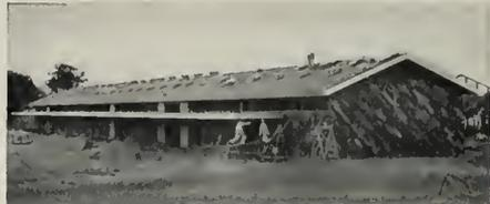
To protect against termite damage for the life of the buildings, BAXCO Chemonited (pressure treated) Lumber was used for sill plates, wall studs, rafters, and sheathing.
