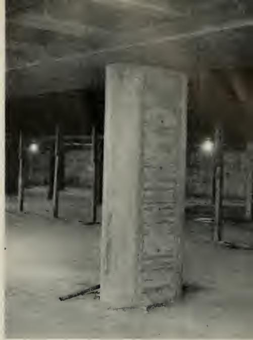
18" x 36" columns from the fourth floor to the fifth floor are smaller to provide wider aisles. NOTE a typical column used elsewhere in the construction is 18" x 54".
