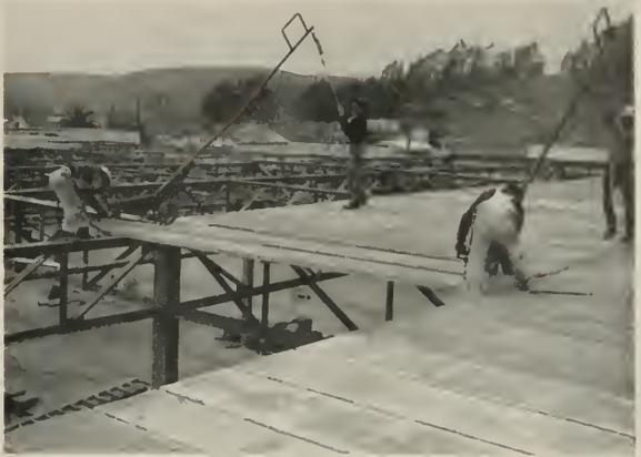
Placement of channel slabs of 20 foot span on girders by crane.
