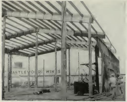
SHOWING erection of prefabricated wall section of United States Products Warehouse in San Jose, California. Walls were raised in 20 ft. sections by fork lift truck.
