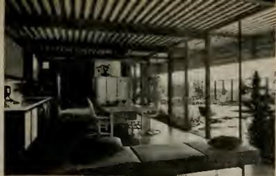
The X-100 was designed to utilize standard United States Steel sections: 4" H13# for vertical columns; 8" WF13# and 10" WF17# for roof beams. There was also a variety of small angles, T's and channels involved. Steel roof decking was fabricated by H. H. Robertson.
