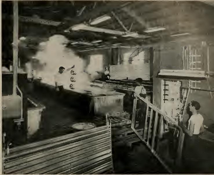
or a rectifier unit supplying 15 to 18 volts of direct current which in turn, will normally produce approximately  $12\frac{1}{2}$  amp. per sq. ft. of work in the bath.
