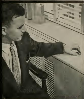
*A unique feature of the Equitable Building's air-conditioning is 1,180 of these air blending units. There is a blender installed in every perimeter office. The units are connected to the central duct system and they act as independent thermostats delivering conditioned air according to an individual's wants.*
