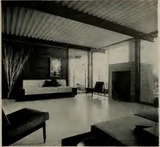
**A STEEL HOUSE FOR MASS PRODUCTION:** In this residence, designed for mass production, Architect Soriano has utilized 10 ft. by 26 ft. module steel, plus a 1½ in. steel decking. I-beams extend beyond walls, with steel sash and floor to ceiling windows, to provide roof extension for shade and protection. Interior has exposed steel beams. (1955)
