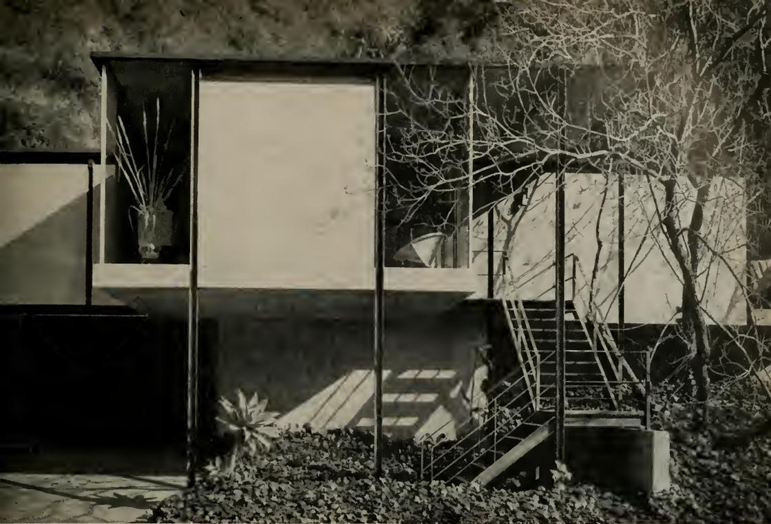
*This home, the first hillside-design created by Ellwood using a modular steel frame, was built in 1952. Today, this 1400 sq. ft. house could be built for about \$12.50 per square foot—including built-in appliances. The owner of this steel-framed home is forever protected against termites as well as warping and checking. Steel is permanent...and needs little upkeep.*
