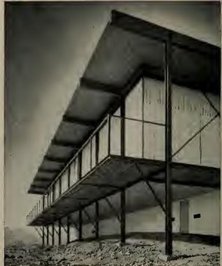
*Craig Ellwood's fifth hillside steel home illustrates how he uses individual concrete pads to eliminate costly continuous footings and allow openness of structure. Floor is supported by 6" 8.2# steel channels. The 1" square bars used for tie rods (diagonal bracing at right) eliminate the need for solid shear walls.*
