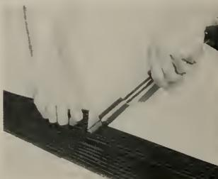
PLASTI-GRIP's deep grooves grip far better into concrete than flat or dumbbell type joints and its exclusive reinforced "U" shaped center pleat expands and contracts with the joint. It is designed to give the most effective joint between two pours of concrete.
