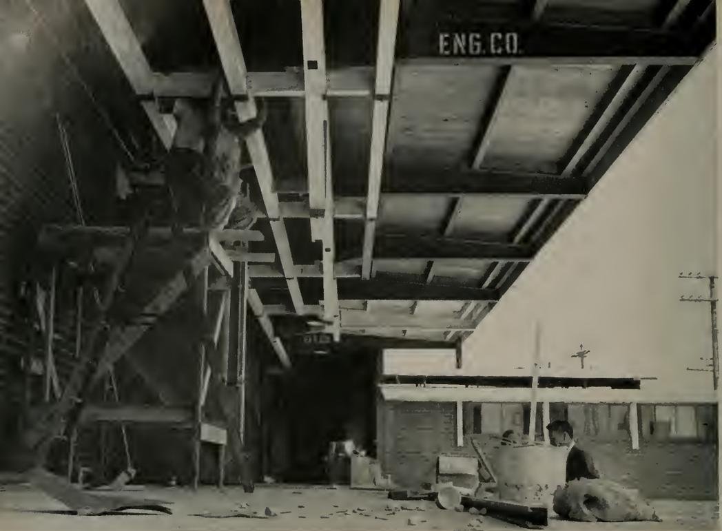
UPPER FOREGROUND shows a section of the 20 x 102 foot overhang. Four by eight foot panels of  $\frac{3}{4}$ -inch tongue and grooved fir plywood used effectively to eliminate cost of expensive blocking at unsupported panel edges.
