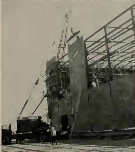
**TILT-UP CONCRETE SLAB** is being hoisted into second floor position for affixing to steel.
