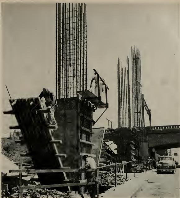
The concrete "legs" for San Francisco's new Embarcadero Freeway are being built with the heaviest steel reinforcing bars ever used in overhead highway construction in California's ever expanding State Highway system.
