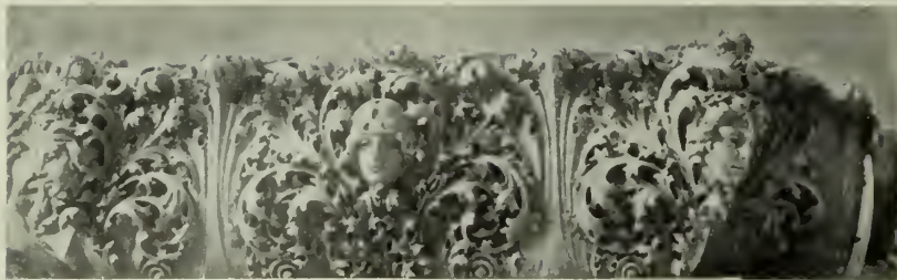
IMPOST CAP, MAIN ENTRANCE, CANTON BUILDING, CLEVELAND, OHIO. Executed by the Northwestern Terra-Cotta Company. F. S. Barnum & Co., Architects.
