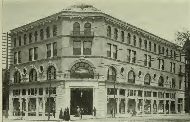
ROWE DEPARTMENTAL STORE, PITTSBURGH, PA. Architectural terra-cotta furnished by the Winkle Terra-Cotta Company, St. Louis. Brick by the New York Hydraulic-Press Brick Company. Alden & Harlow, Architects.
