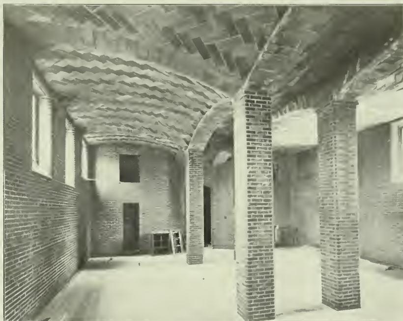
FINISHED ROUGH TILE CEILINGS AND FLOORS, MASSACHUSETTS GENERAL HOSPITAL BUILDING, BOSTON.
