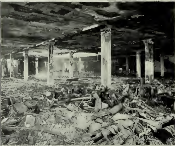
FIG. 6. FIFTH STORY LOOKING NORTHEAST. CONTENTS BURNED OUT EXCEPT ROLLS OF CARPET NEAR THE FRONT.
