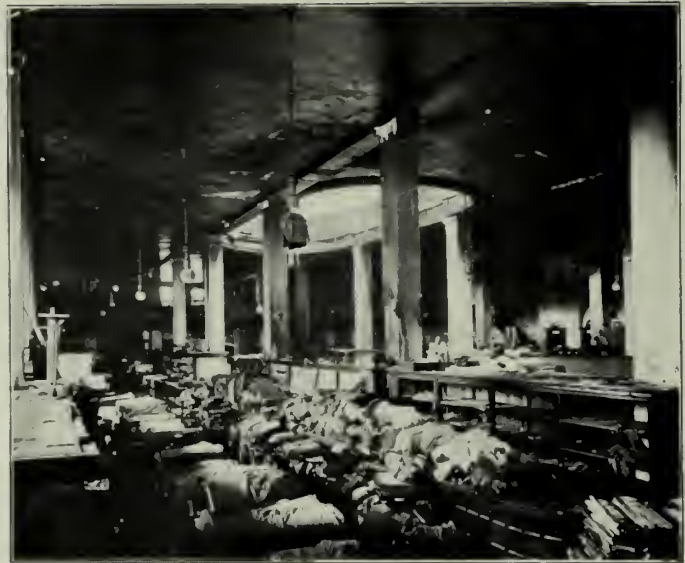
FIG. 1. FIRST STORY LOOKING NORTH, SHOWING DAMAGE BY SMOKE AND WATER ONLY. THE SMOKE AND HOT AIR CAME FROM FIRE IN BASEMENT.
