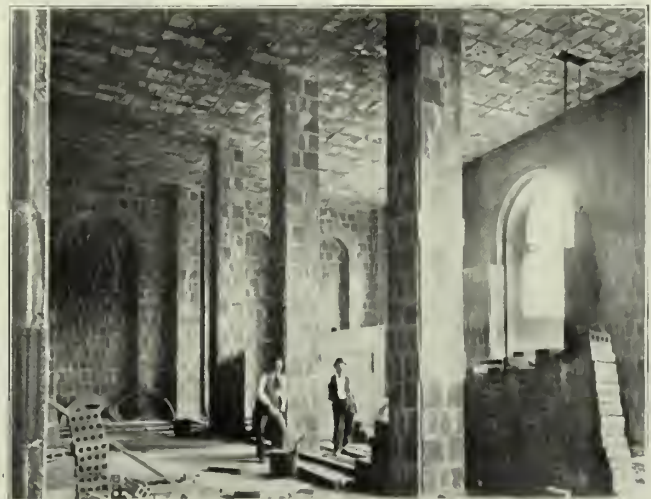
Terra-Cotta Fire-proof Construction. NEW PRUDENTIAL BUILDINGS, NEWARK, N. J. Executed by the Raritan Hollow and Porous Brick Co. George B. Post, Architect.
