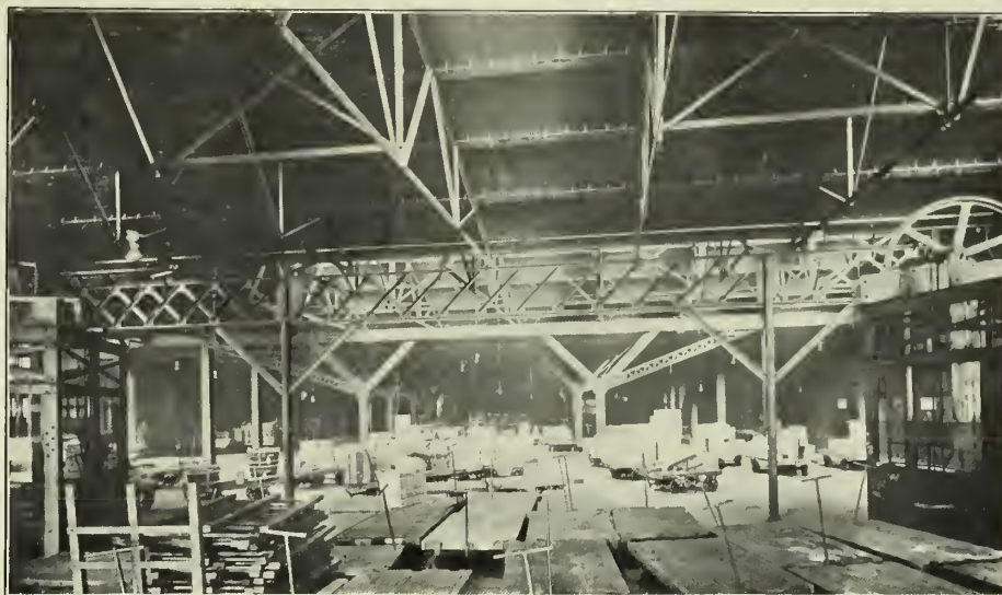
FIG. 2. UPPER LEVEL SHIPPING PLATFORM, SHOWING TRIANGULAR TRUSSES IN BACKGROUND.
