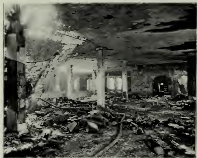
FIG. 8. SIXTH STORY LOOKING SOUTHEAST, SHOWING KITCHEN PARTITION WHICH SAVED COOKING APPARATUS, AND CEILING FALLEN ON THE LEFT.
