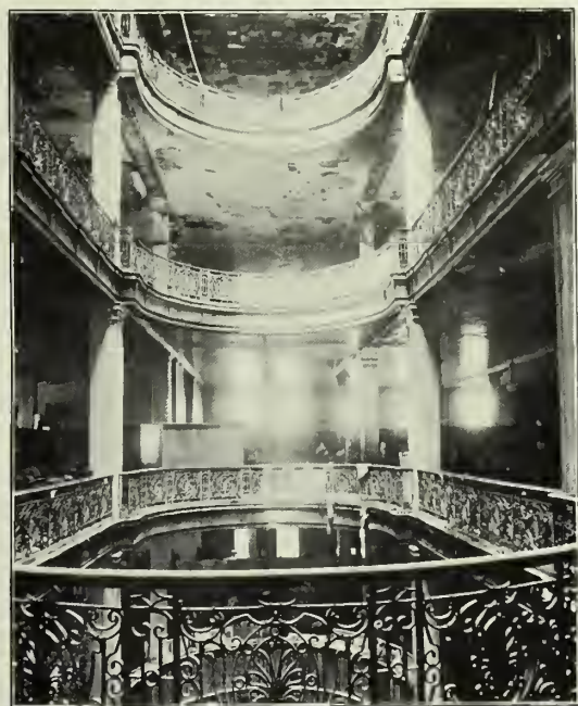
FIG. 3. THIRD STORY, SHOWING FOURTH AND FIFTH ABOVE AND FIRST STORY BELOW LOOKING NORTH. THIS FLOOR ONLY DAMAGED BY WATER.
