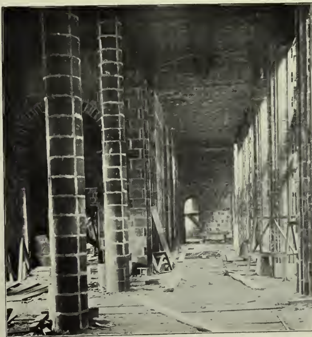
TERRA-COTTA FIRE-PROOF CONSTRUCTION, CITY POST OFFICE, WASHINGTON, D. C. Work done by the Central Fire-proofing Company.
