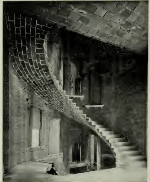
FIG. 21. ELLIPTICAL STAIRWAY, FIRST NATIONAL BANK, PATERSON, N. J.
