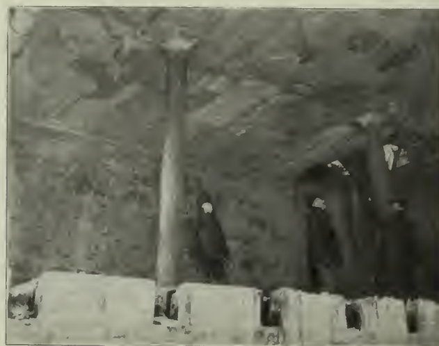
FIG. 1. SHOWING PROTECTION TO SOFFIT OF GIRDERS AND HOW IT RESISTED ONE OF THE HOTTEST FIRES ON RECORD.
