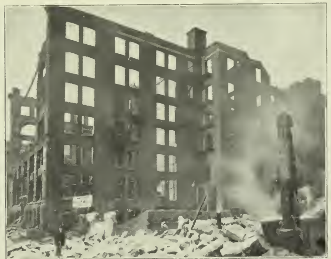
SHOWING COMPARATIVE EFFECT OF A FIERCE FIRE ON A STONE AND A BRICK WALL.
