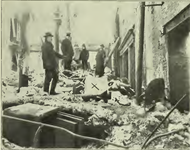
FIG. 2. SHOWING LOAD ON TERRA-COTTA FLOOR. AT RIGHT, REMAINS OF A TIN-COVERED DOOR X SAFE, FALLEN FROM ABOVE.
