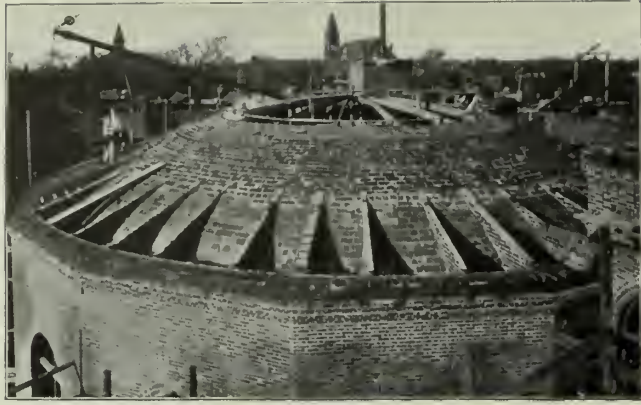
FIG. 5. DOME, EAST BOSTON HIGH SCHOOL, 70 FEET DIAMETER.
