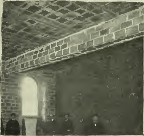
TERRA-COTTA FIRE-PROOF CONSTRUCTION, FREE PUBLIC LIBRARY BUILDING, NEWARK, N. J. Work executed by the Raritan Hollow and Porous Brick Company. Rankin & Kellogg, Architects.
