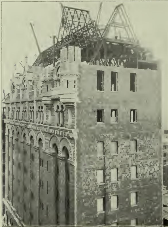
PRUDENTIAL BUILDING, NEWARK, N. J. Showing wall built of hollow tile fire-proof blocks. Raritan Hollow and Porous Brick Company, makers. George B. Post, Architect.
