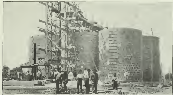
FIG. 7. TANKS OF NORTH STAR MALTING COMPANY, MINNEAPOLIS, IN PROCESS OF CONSTRUCTION.
