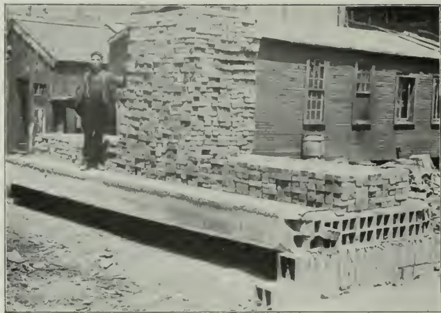
FIG. 1. TEST OF JOHNSON SYSTEM OF FLOOR CONSTRUCTION AT AKRON, OHIO, JULY, 1898.
