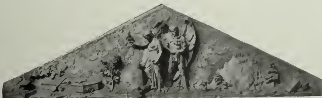
47 FEET LONG, 11 FEET HIGH. TYMPANUM EXECUTED IN TERRA-COTTA BY EXCELSIOR TERRA-COTTA COMPANY. J. Mills Platt, Architect.
