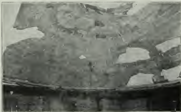
UPPER FLOOR, PATERSON SAVINGS INSTITUTION, SHOWING GUASTAVINO TILE DOME AFTER FIRE. WHITE PATCHES SHOW PLASTER ON TILES.
