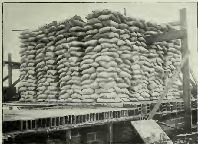
FIG. 3. PUBLIC TEST OF JOHNSON FLOOR CONSTRUCTION MADE AT MINNEAPOLIS, AUG. 7 9, 1901, AS REPORTED BY PROF. W. R. HOAG.
