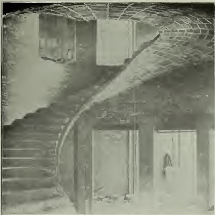
GUASTAVINO SPIRAL STAIRCASE. CONSTRUCTION FOR MAIN STAIRS, UNION CLUB, NEW YORK CITY. Cass Gilbert and John Du Fais, Associate Architects.
