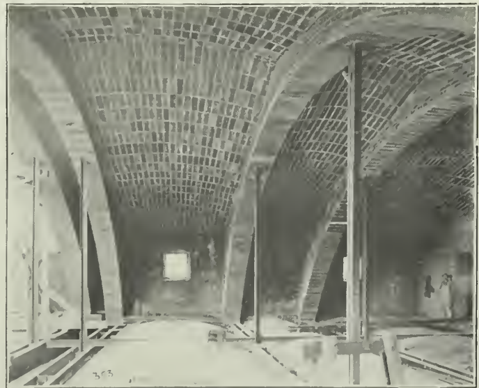
VIEW OF MASONRY ROOF GIRDERS AND ROOF AND FLOOR CONSTRUCTION OF STABLE FOR HOWARD GOULD, ESQ. BUILDING ABOUT FOUR HUNDRED FEET LONG. GUAUSTAVINO CONSTRUCTION THROUGHOUT.
