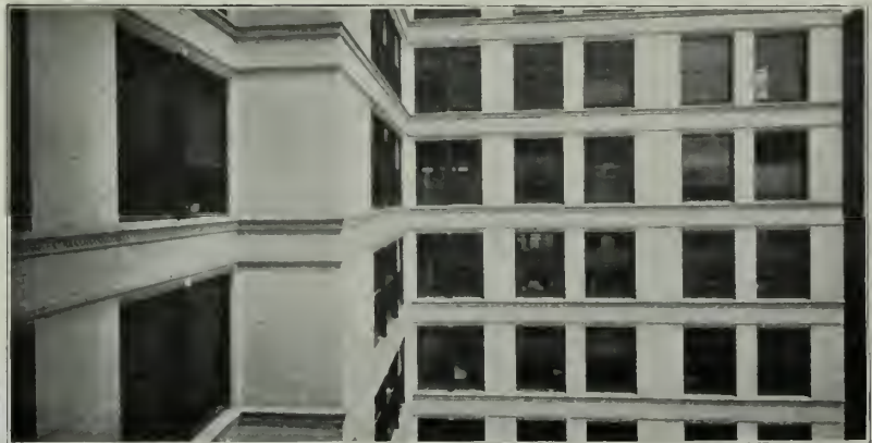
COURT OF OFFICE BUILDING, SHOWING USE OF ENAMELED BRICK. Made by Tiffany Enameled Brick Co.
