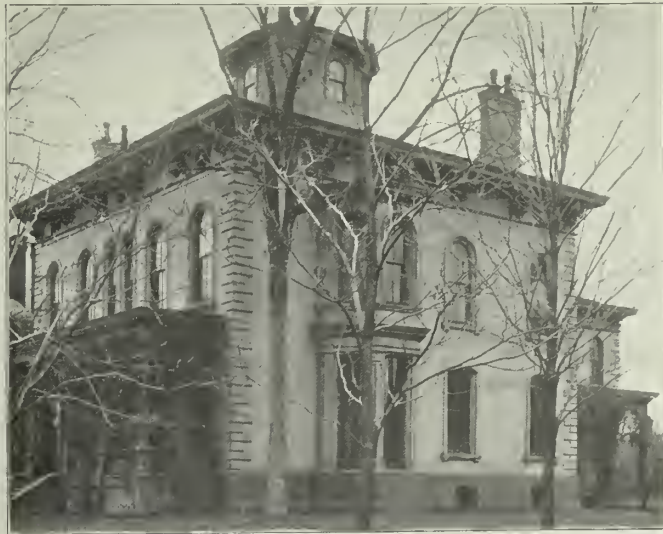
HOUSE AT BUFFALO, MONOLITH CONSTRUCTION. BUILT IN 1870.
