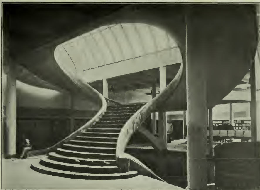
GRAND STAIRCASE, GUASTAVINO CONSTRUCTION. DEPARTMENT STORE, PATERSON, N. J. Treads and risers ready to receive finish.
