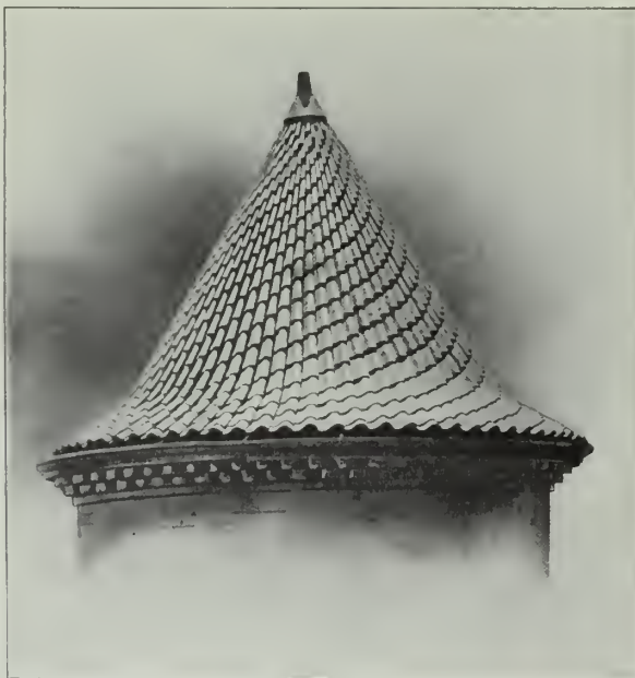
SHOWING METHOD OF PUTTING ON GRADUATED AMERICAN "S" TILE ON CIRCLE ROOFS AND TOWERS. EACH TILE IN EACH COURSE IS GRADUATED FROM GUTTER TO APEX TO FORM A PERFECT RADIATION.
