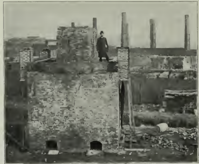
"NEW YORK" REINFORCED TERRA-COTTA ARCH, SHOWING PILE OF BRICK EQUAL TO SIX HUNDRED POUNDS PER SQUARE FOOT OVER ARCH SIX FEET BY FOURTEEN FEET, CARRIED BY THE ARCH AFTER THE FIRE AND WATER TEST. NOTE CRACK IN TEST HOUSE WHICH CAUSED THE SPREADING OF THE BEAMS.
