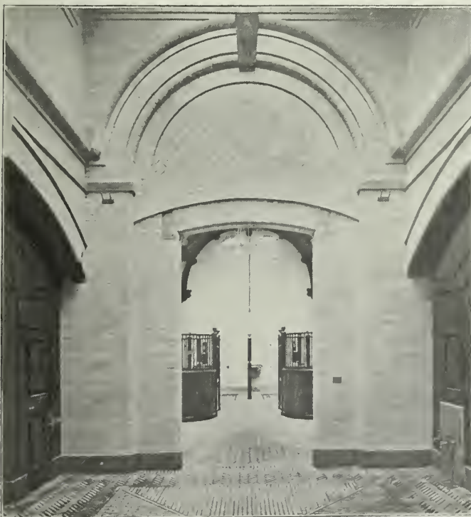
INTERIOR OF STABLE, SHOWING USE OF BLUE RIDGE ENAMEL BRICK, CREAM TINT. Warren & Wetmore, Architects.
