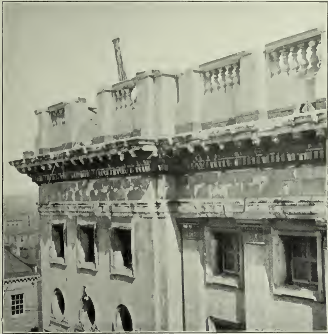
CORNICE OF THE NEW COURTHOUSE, SHOWING DAMAGE TO THE MARBLE.
