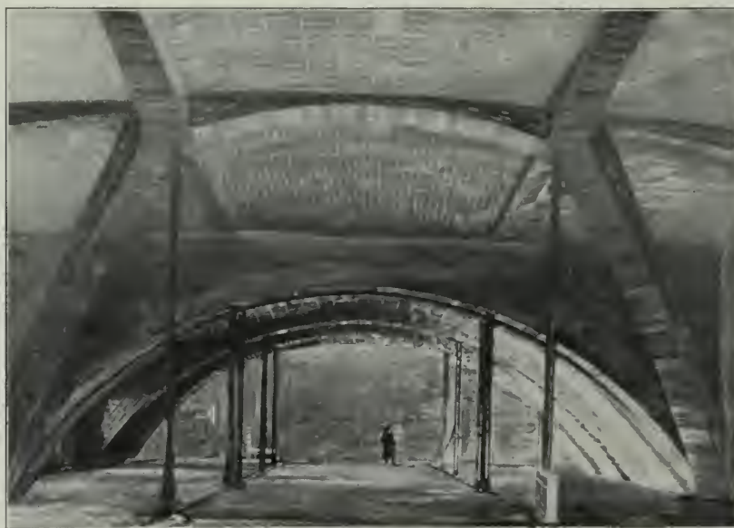
STABLE FOR HOWARD GOULD, ESQ., PORT WASHINGTON, L. I. View of roof construction showing supporting masonry ribs and hangers from same, partially carrying floor below. Spans about 50 feet. Guastavino construction.
