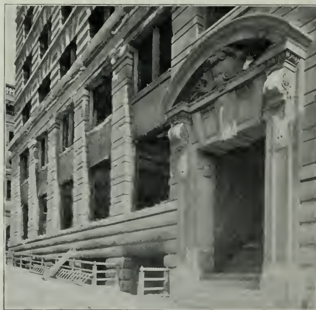
DETAIL, CALVERT BUILDING, SHOWING BADLY SPALLED STONE.
