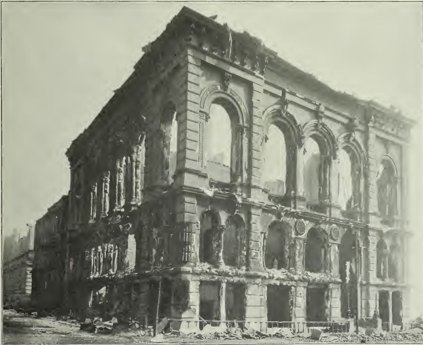
THE RIALTO BUILDING, SHOWING THE EFFECT OF FIRE ON STONE.
