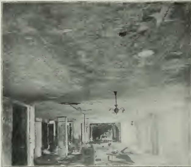
VIEW OF THE FIRST FLOOR OF THE CONTINENTAL TRUST BUILDING, SHOWING THE EFFICIENCY OF THE FIREPROOFING.
