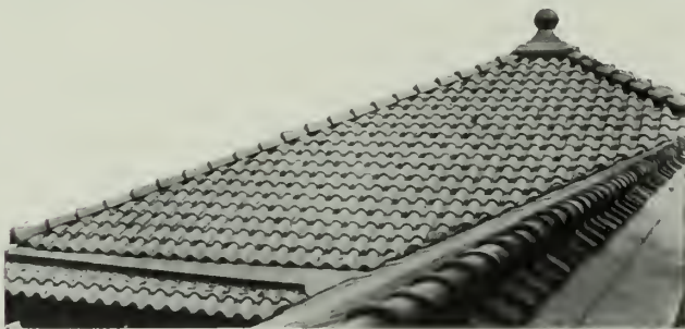
ROOF OF A BUILDING IN PITTSBURG, ON WHICH FOLSOM SNOW GUARDS ARE USED IN COMBINATION WITH TILE.
