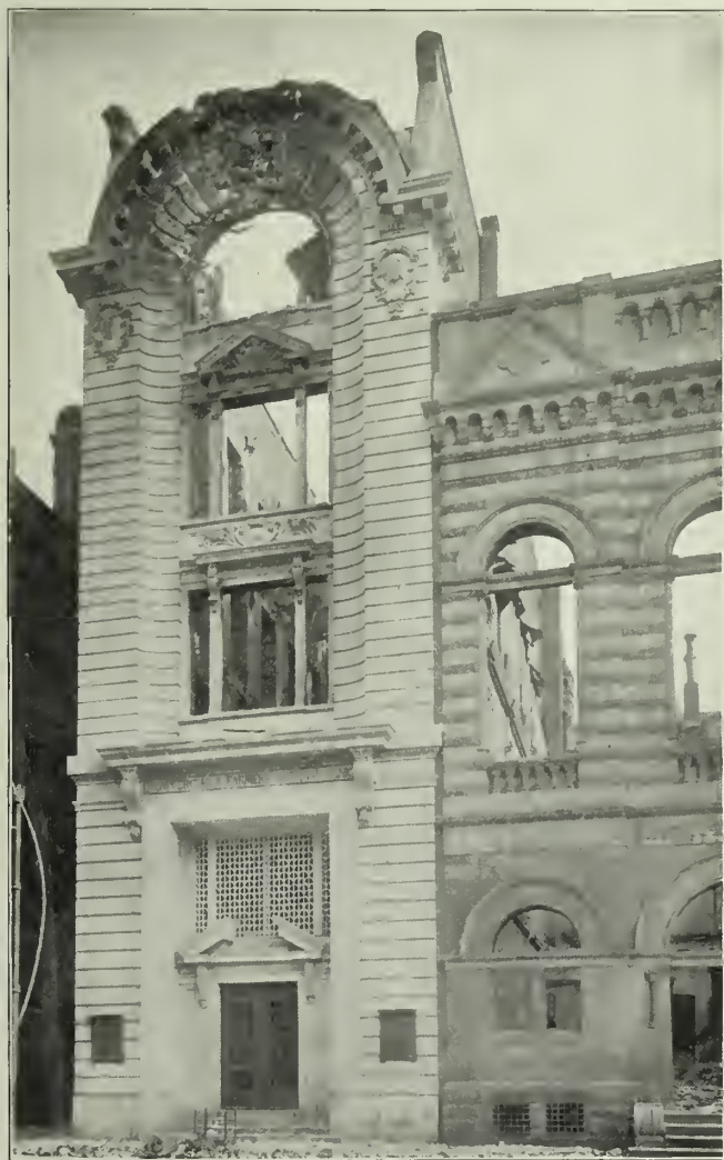
THE COMMERCIAL AND FARMERS' NATIONAL BANK BUILDING. Wyatt & Nölting, Architects. Showing damage to stone where licked by flame.
