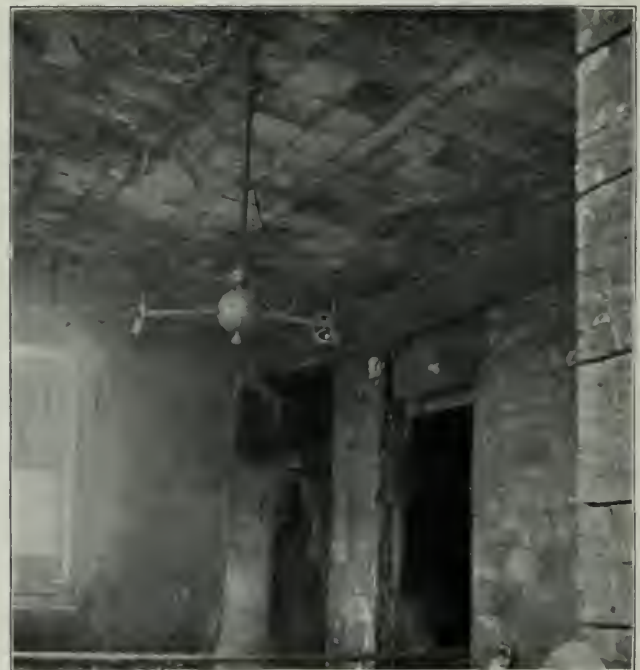
A ROOM IN THE MERCHANTS' NATIONAL BANK BUILDING, SHOWING PERFECT CONDITION OF THE FIREPROOFING.
