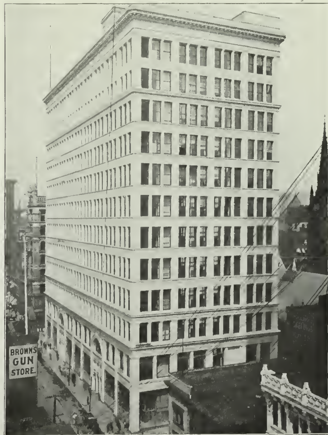
OLIVER BUILDING, PITTSBURG, PA. D. H. Burnham & Co., Architects. Built of white enameled terra-cotta, made by Northwestern Terra-Cotta Co. Fireproofed by the National Fireproofing Co.
