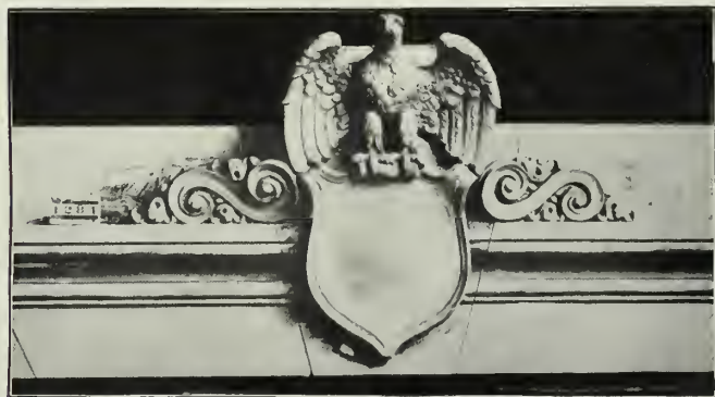
DETAIL FOR WINDOW HEAD. R. Thomas Short, Architect. New Jersey Terra-Cotta Co., Makers.
