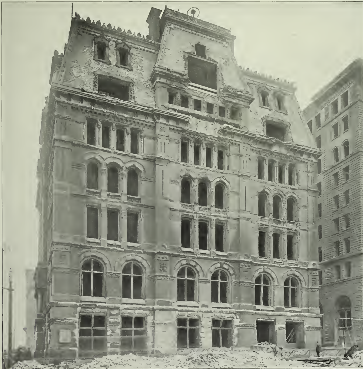
BALTIMORE AND OHIO BUILDING. Showing utter ruin of stone trim around openings.
