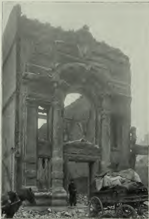
HAMBLETON & COMPANY'S BANK BUILDING, SHOWING THE EFFECT OF FIRE ON LIMESTONE.
