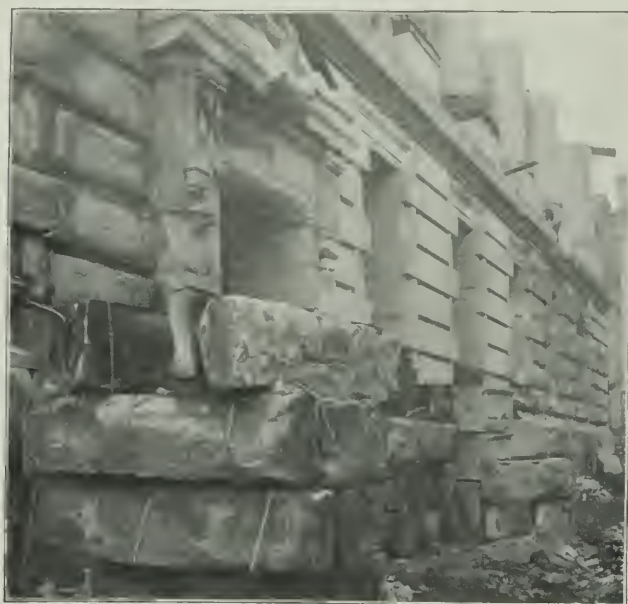
GRANITE ON GROUND AT CUSTOM HOUSE, BADLY SPALLED, THOUGH HEAT NOT INTENSE.
