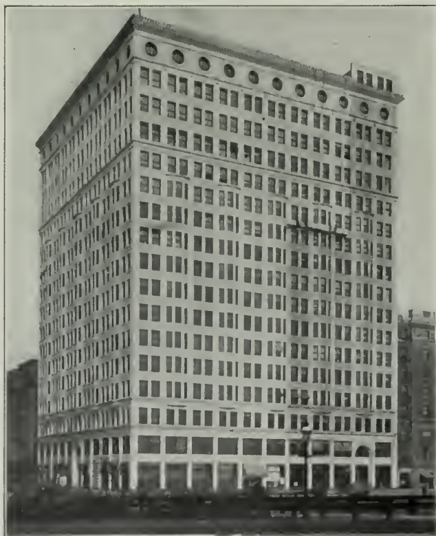
AN ENAMEL FINISH TERRA COTTA "SKYSCRAPER" BEING GIVEN ITS ANNUAL BATH. THERE ARE ABOUT 200,000 SQUARE FEET OF EXTERIOR SURFACE WHICH IS WASHED EVERY SPRING AT A COST OF $1,000.
