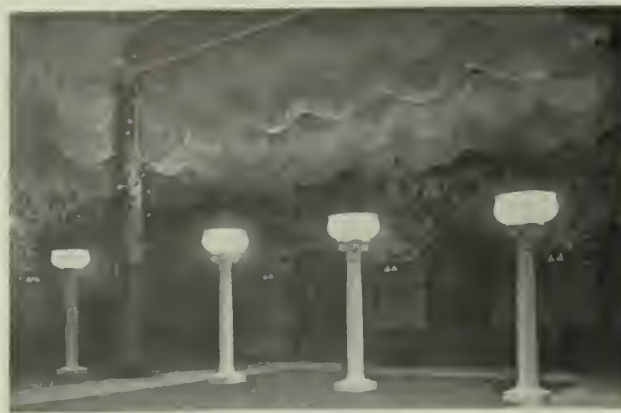
FIG. XXVIII. SPECIAL SEMI-INDIRECT GAS LIGHTING INSTALLATION AT TAFT HALL, AUDITORIUM ARMORY, ATLANTA, GA.
