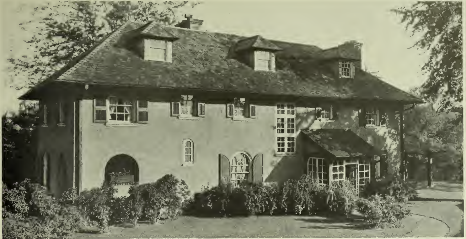
HOUSE AT ST. MARTINS, PA. (EXTERIOR WALLS OF TERRA COTTA HOLLOW TILE) EDMUND B. GILCHRIST, ARCHITECT
