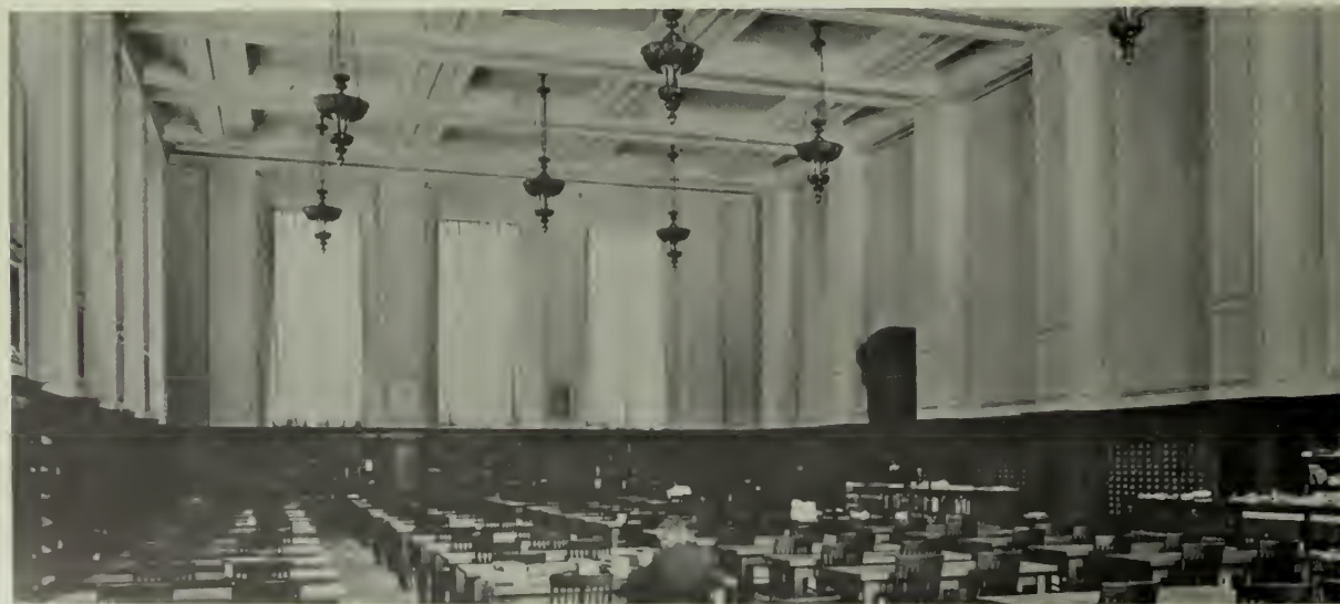
FIG. XVII. INDIRECT LIGHTING INSTALLATION IN READING ROOM, JOHN HAY'S MEMORIAL LIBRARY, PROVIDENCE, R. I.
