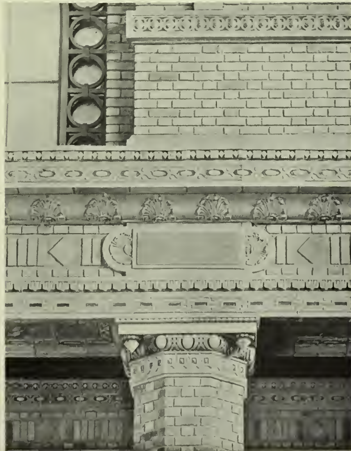
DETAIL OF COLUMN AND ENTABLATURE
