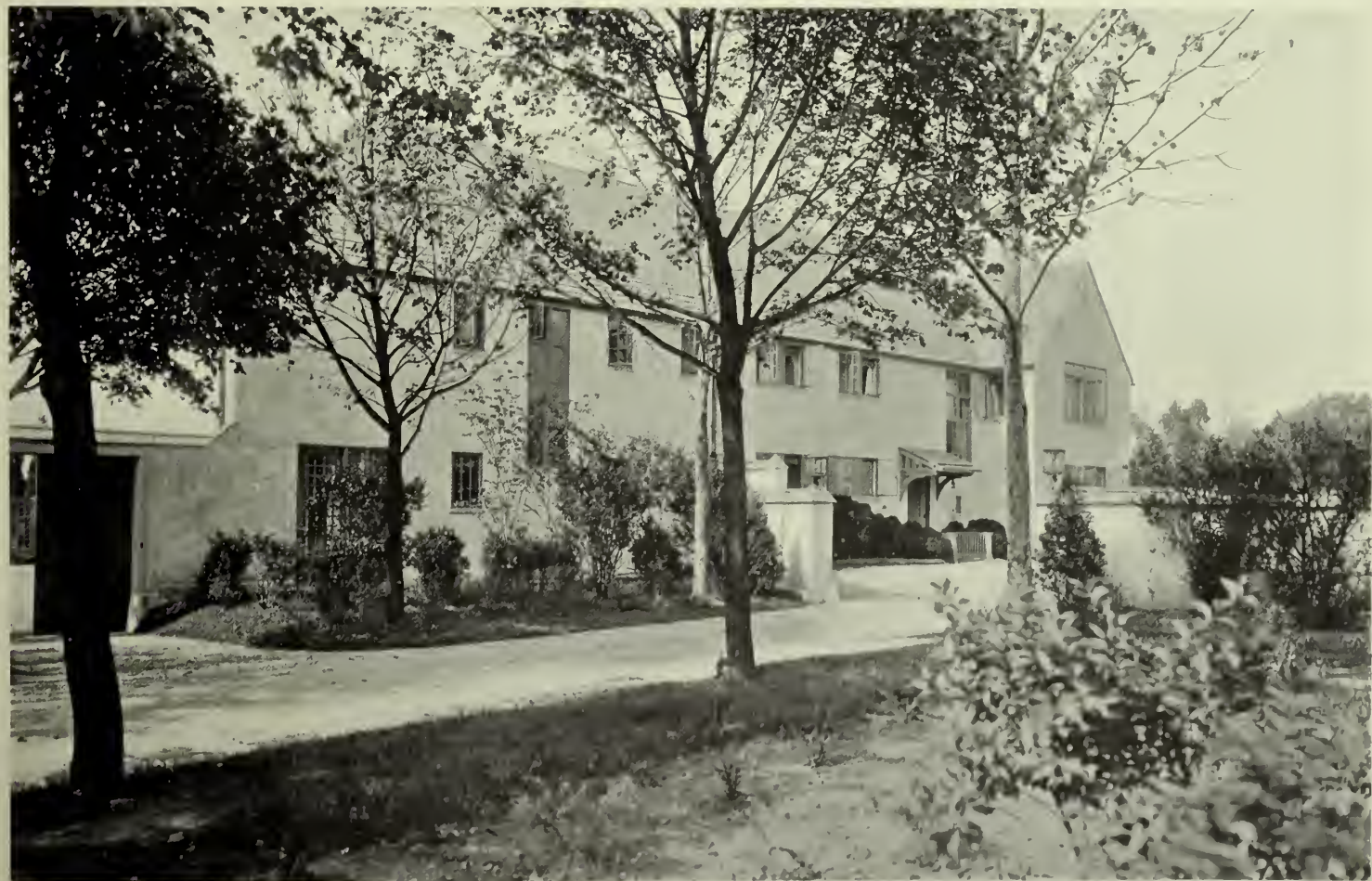
HOUSE AT BERNARDSVILLE, NEW JERSEY EXTERIOR WALLS OF TERRA COTTA HOLLOW TILE DELANO & ALDRICH, ARCHITECTS
