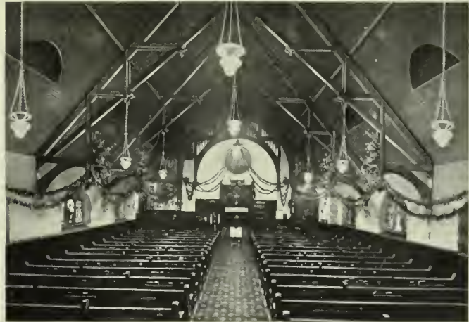
FIG. XXXIII. DIRECT LIGHTING INSTALLATION IN CHURCH AT SEWICKLEY, PA.
