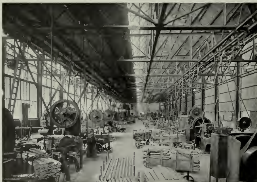
Method Combining Advantages of Sawtooth Roof and Lantern Lighting and Ventilation
