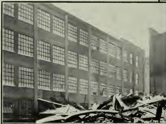
Fenestrated Factory of The Reliance Gauge Column Co., Cleveland, Ohio. C. N. Griffin Co., Contractors. The small photo above shows the complete destruction of the wooden factory closely adjoining the Fenestrated Reliance Gauge Column Co.'s building. Note in photo at right how the brick and concrete were scaled by the intense heat.
