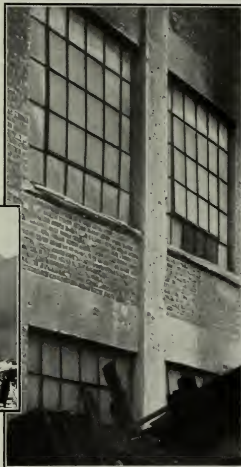
Fenestrated Factory of The Reliance Gauge Column Co., Cleveland, Ohio. C. N. Griffin Co., Contractors. The small photo above shows the complete destruction of the wooden factory closely adjoining the Fenestrated Reliance Gauge Column Co.'s building. Note in photo at right how the brick and concrete were scaled by the intense heat.
