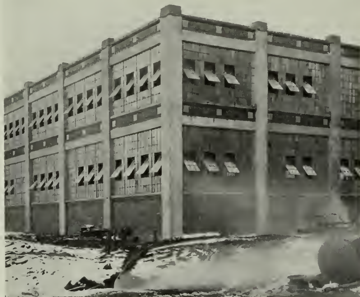
In Very Wide Buildings it Is Necessary to Diffuse the Light Admitted so as to Reach and Evenly Illuminate the Central Portions of Work Rooms
