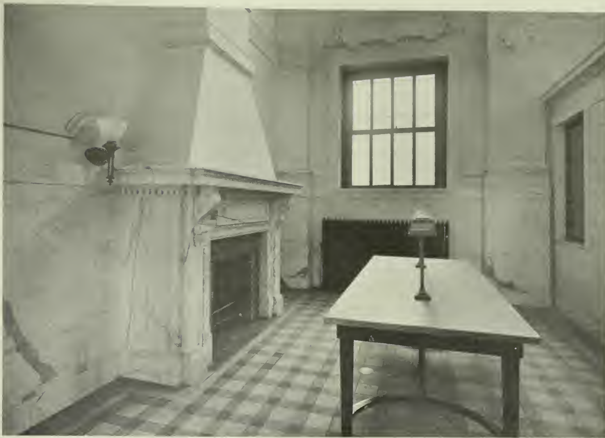
This Linotile floor, in the directors' room of the German Bank, Louisville, Ky., is composed of 6" x 6" white, 3" x 6" light gray and 3" x 3" dark gray tile. D. X. Murphy & Brothers, Architects, Louisville, Ky.
