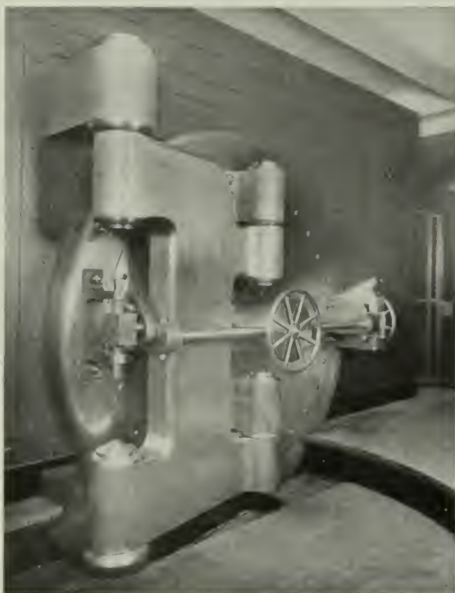
Exterior View of Fifty-ton Door Note movable platform in lower position
