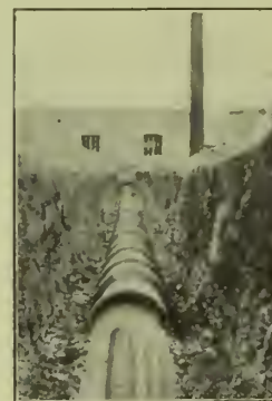
Installing J-M Sectional Conduit at State School of Mines, Rapid City, So. Dak.
