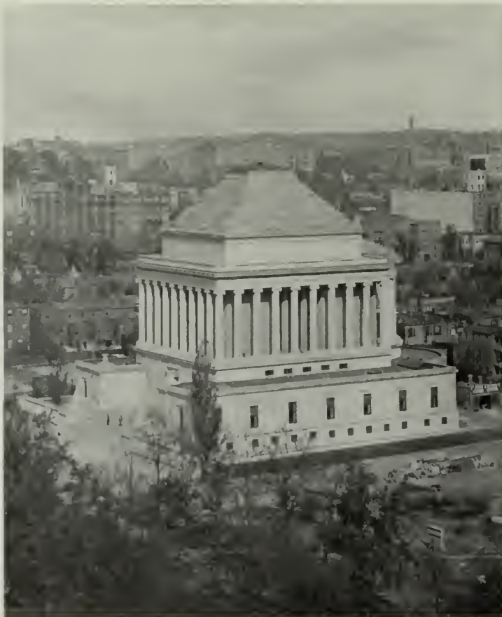
View of Building, Showing Solid Limestone Roof
