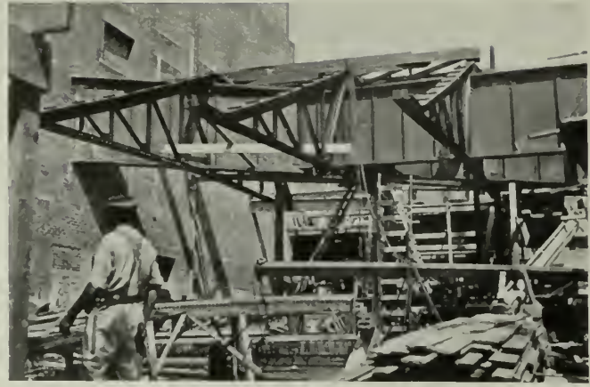
View Showing Cantilever Balcony Trusses
