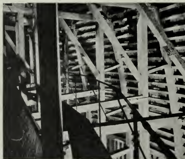
Dome of St. Paul's, London. View Between Brick Cone and Outer Dome
