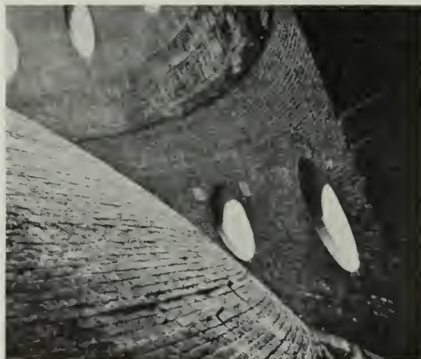
Dome of St. Paul's, London. View Between Inner Shell and Brick Cone
