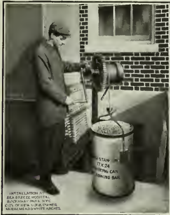
One man, unaided, can perform entire operation of raising filled cans to sidewalk and lowering empty cans to cellar.
