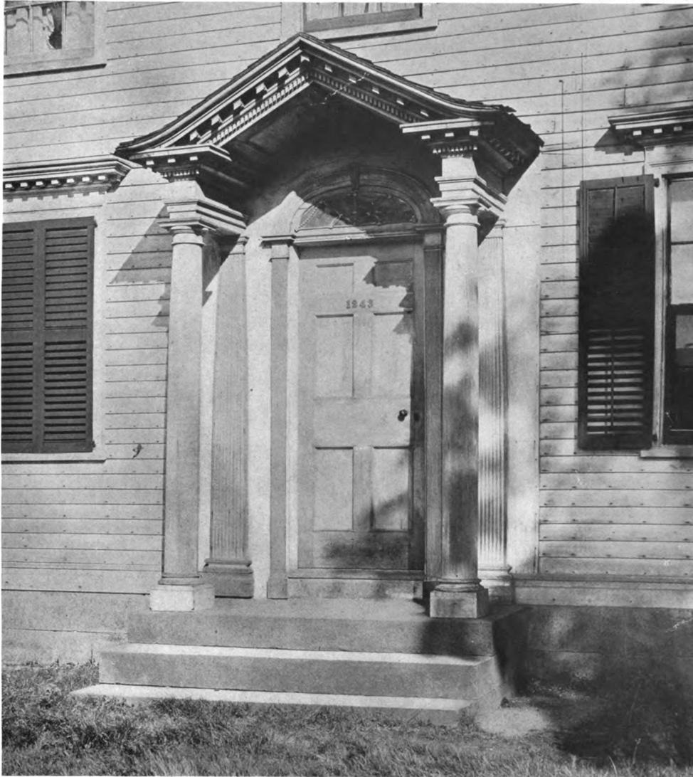
*THIS* entrance is built of white pine, except the shafts of the columns, which are turned from solid pieces of maple. Its most pleasing feature, perhaps, is the curve with which the sloping roof terminates on either side. This is repeated in the main cornice of the house at the ends of the gables.
