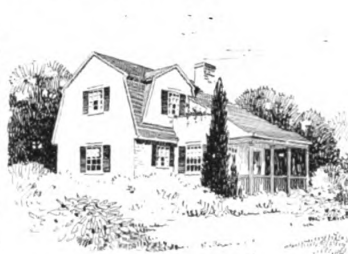
Single Cottage with Floor Plans at Right. Frame and Shingle Construction. Bathroom. Heated by Stoves.
