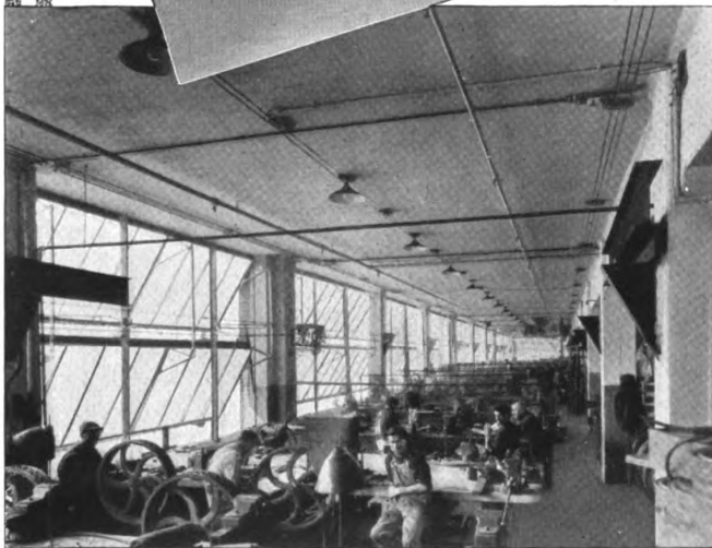
Firestone Tire & Rubber Company, Akron, Ohio, Mechanical Building; Osborn Engineering Co., Engineers. Pond Continuous Sash gives abundant ventilation without allowing rain to damage goods in process. Note the inside columns, also rail at top of building for hanging window cleaners' swings.
