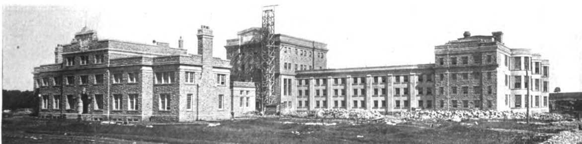
The New Canadian Prison at Guelph, Under Process of Construction This was built almost entirely by the inmates who cast the concrete blocks of which it is constructed
