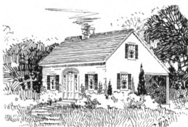
Single Cottage with Floor Plans at Left. Frame and Shingle Construction. Toilet. Heated by Stoves.
