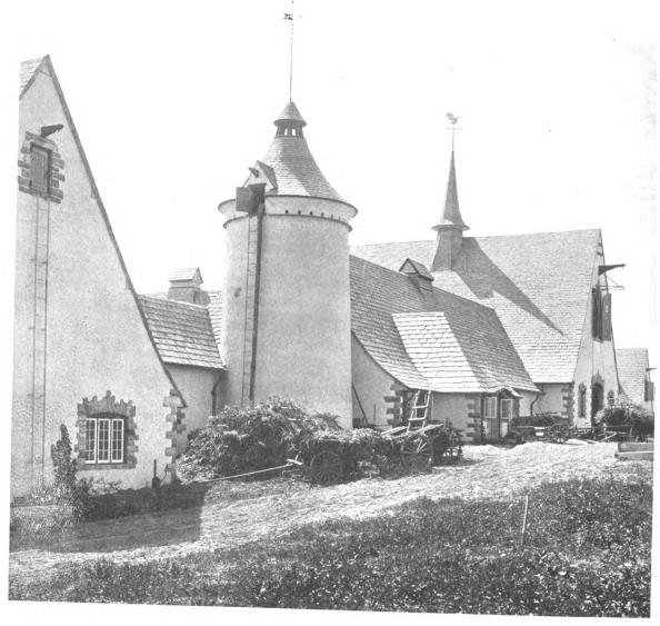
per cent. The height is usually about two and one-half to three times its diameter. The floor should be of concrete and connected to a drain. On account of the odor of the ensilage, it is advisable to have the silo separated from the building or feed
