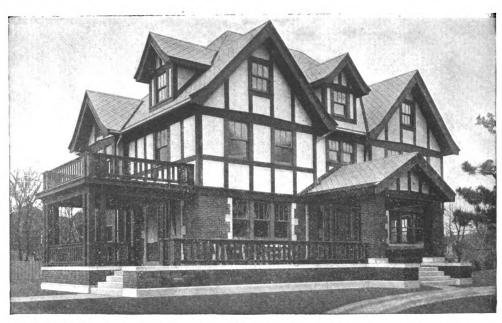
Roof covered with Ambler Asbestos Shingles (Century Brand)—French method. Upper sidewalls covered with Ambler Asbestos Building Lumber—Half-timber effect
