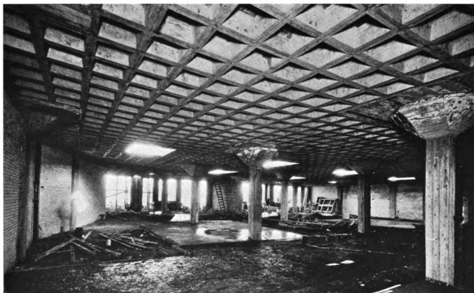
Construction View of Garage Showing Grid Floor System
