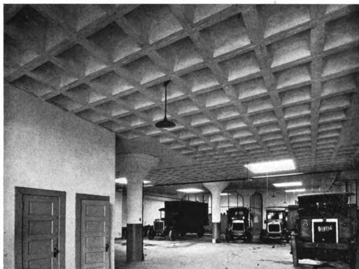
Detail View of Garage Showing Grid System of Floor Construction
