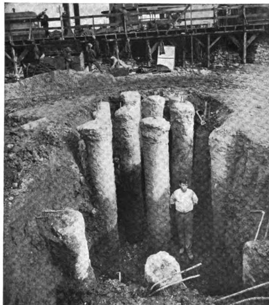
Fig. 1. Concrete Piles Withdrawn for Exposure Test
