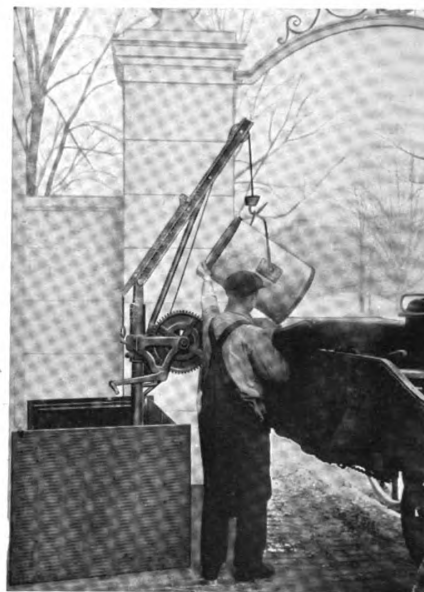
Model B, manually operated G & G Hoist at Phoenix Ins. Co. Bldg., Hartford, Conn. B. W. Morris, Architect. That part of Hoist shown telescopes below grade when not in use.
