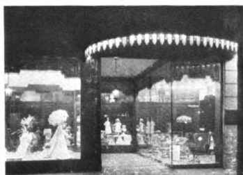
Holophane Installation Reflector Type No. 983
