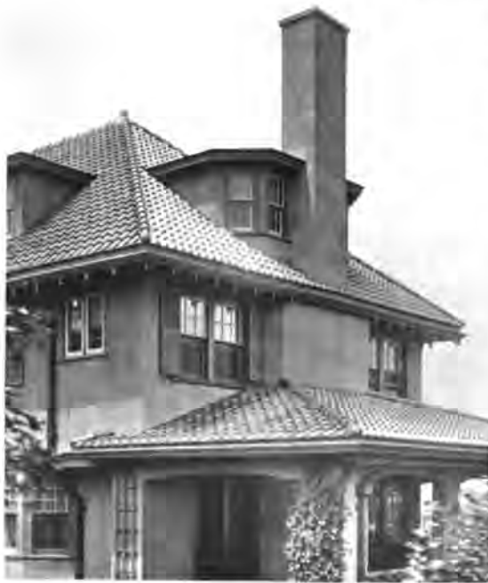
Roof of Spanish or Old Mission Tile Showing Usual Practice in Sloping from Vertical Walls
