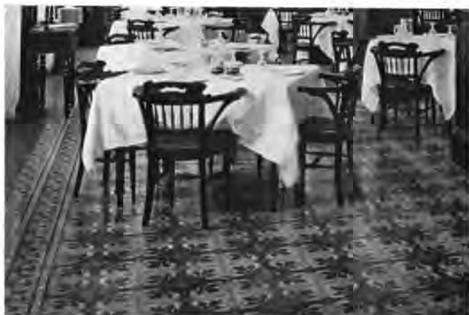
Cement Tile Floor in Pasaje Hotel, Havana, Cuba Each unit is composed of four similar tile
