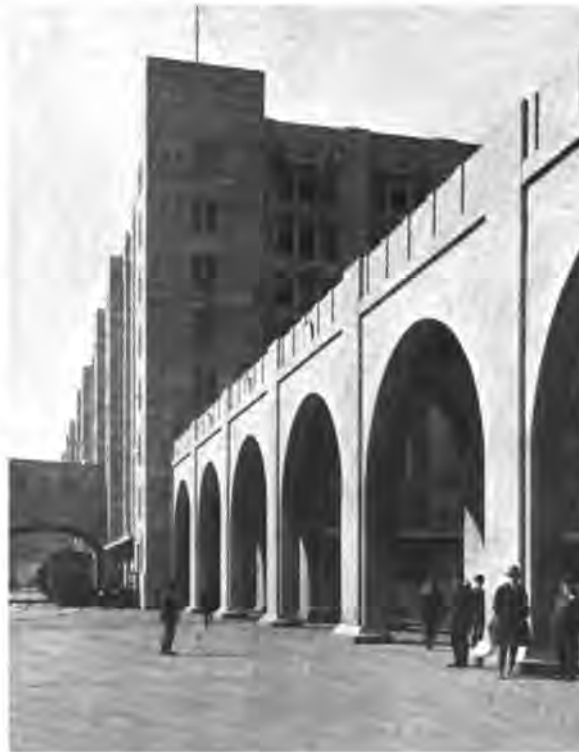
Detail of Connecting Bridges at U. S. Army Supply Base, Brooklyn, N. Y. All Detail in Structural Concrete Cass Gilbert, Architect
