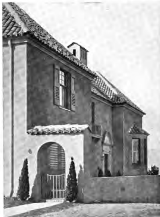
Details of Tile Roofs on Two Houses in California
