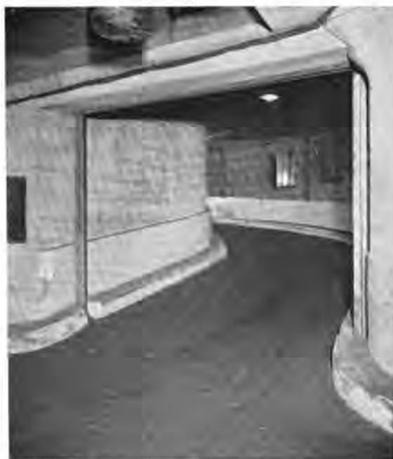
Start of Ramp in LaSalle Garage Showing Fire Door Holabird & Roche, Architects
