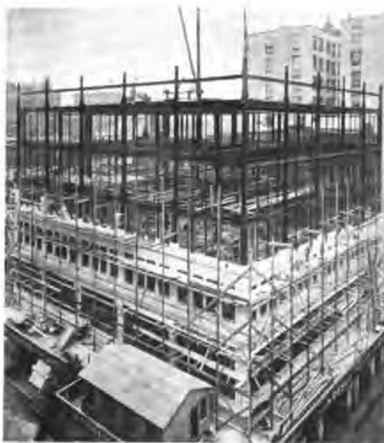
The S. S. Kresge Co. Building, Boston, is Typical Steel Frame Construction, Referred to in this Series of Articles
