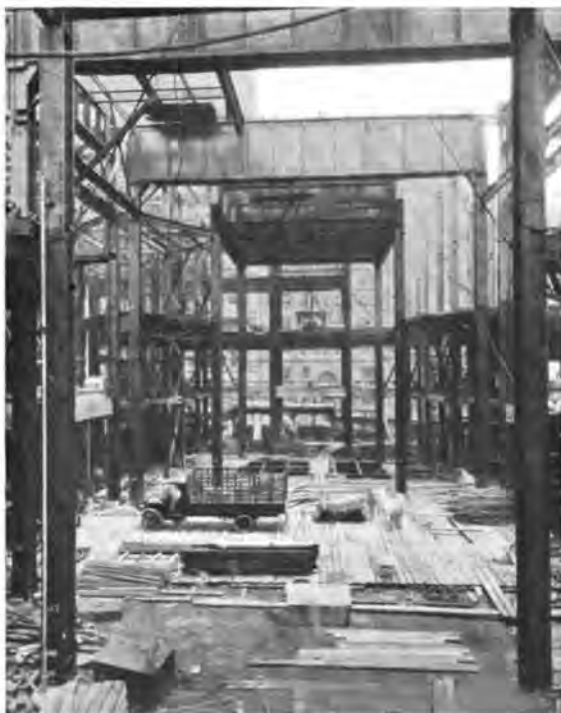
Showing 120-inch Plate Girders in Place
