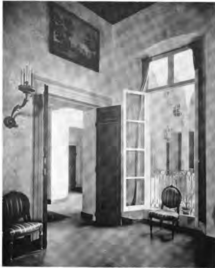
Doorway with Moulded Cement Architrave and Wood Paneled Doors in Italian Style Bigelow & Wadsworth, Architects
