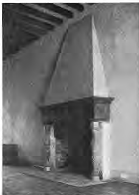
Fireplace in Washington Mews, New York Eric Gugler, Architect Cement columns uphold cornice of unfinished walnut; plaster on walls and between joists
