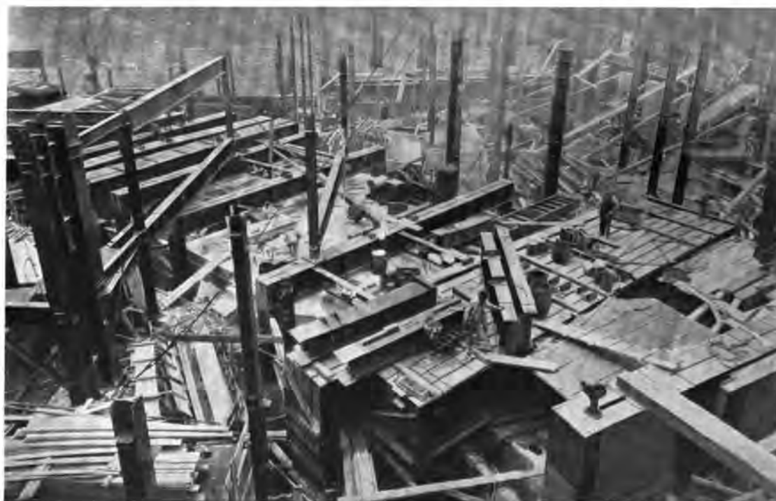
Nine Girders in Foreground over Subway Carry Concentrated Load of 4,200 tons
