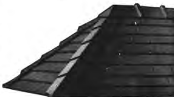
Fig. 3. Closed Shingle Tile with Hip and Ridge
