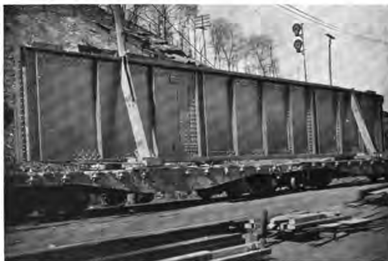
120-inch Plate Girder for Fifth Floor of Cunard Building, Weighing 60 Tons (Fig. 6)
