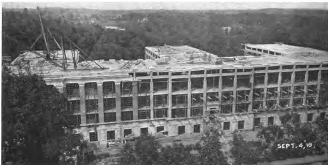
Construction Progress View of Bureau of Standards Laboratory Showing Concrete Frame Completed and Brick and Stone Facing Being Applied Donn & Deming, Architects
