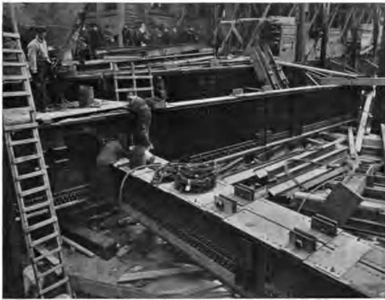
Detail of Framing over Subway Structure Near Greenwich Street Hitch Angles May Be Seen on Tops of Girders
