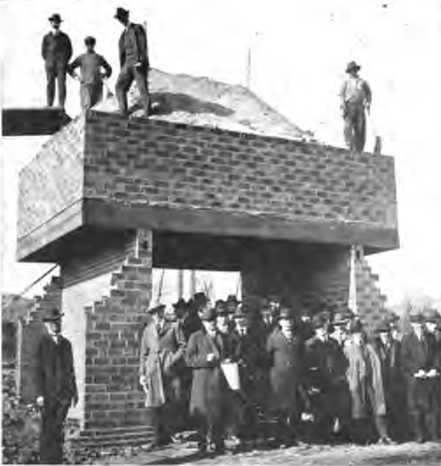
Structural Test, Showing Variety of Bonds
