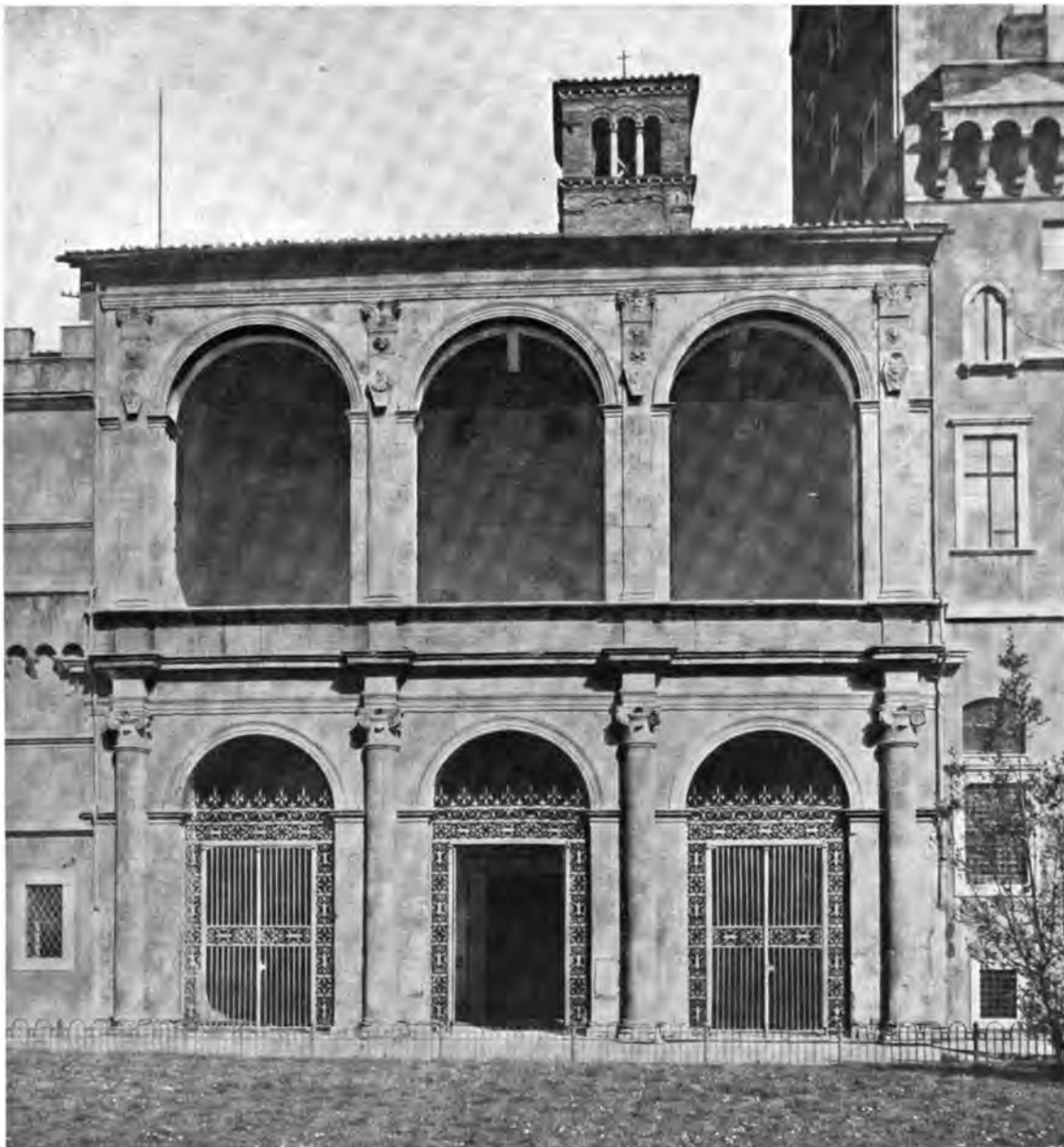
Facade of the Church of St. Mark, Part of the Palace of Venice After the Walls Closing the Arches of the Loggia Had Been Removed
