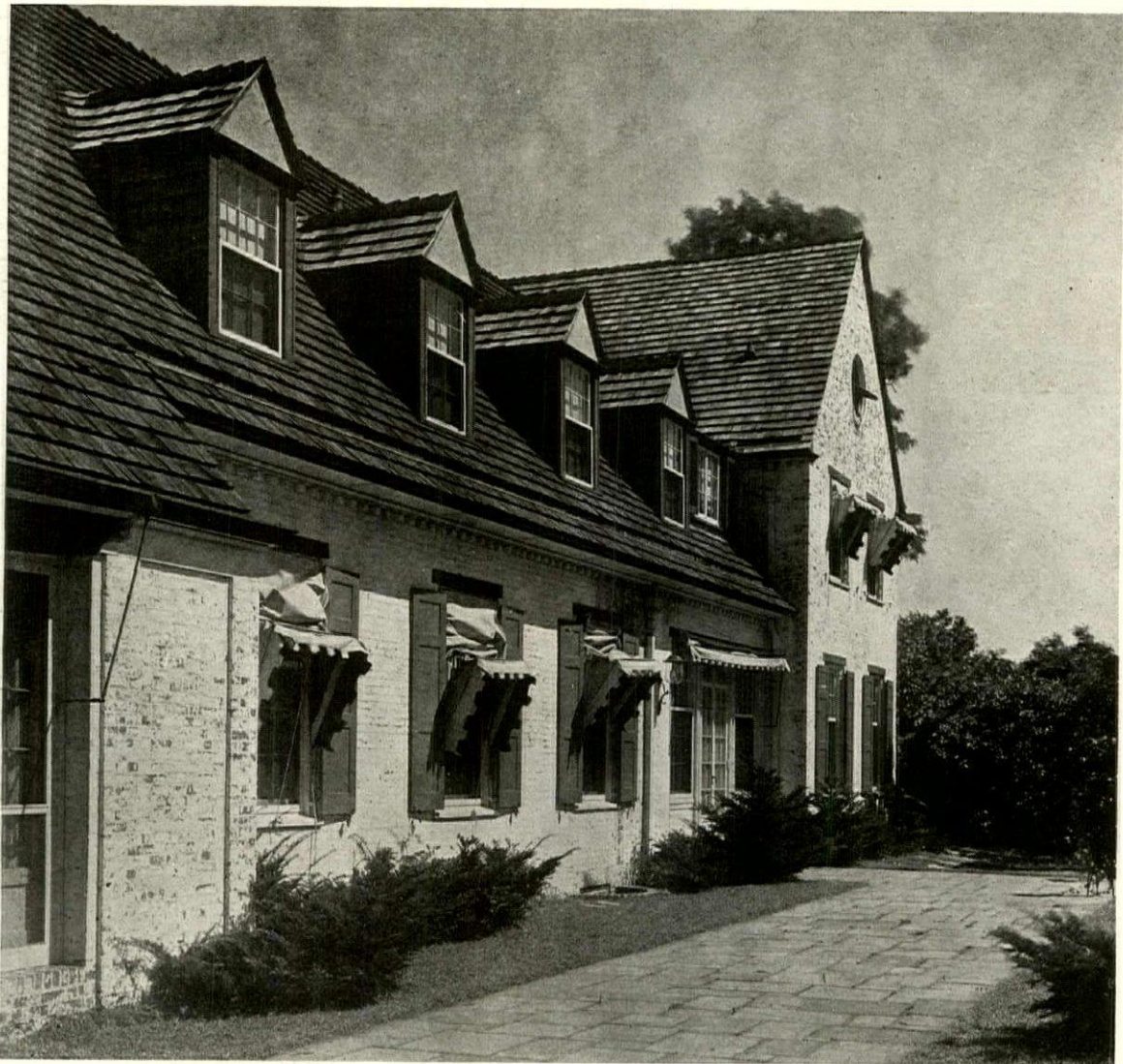
Ordinary building materials handled in manner to secure the utmost effect in color and texture. Walls of whitewashed brick, roofs of cypress shingles, lintels of dark stained oak, flag-paved terrace.
