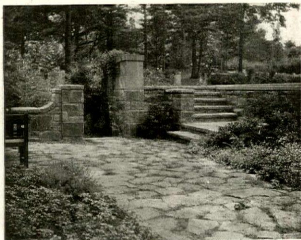
Garden at Wenham, Mass. Stone retaining walls, steps and flag paved paths at intersection of three levels
