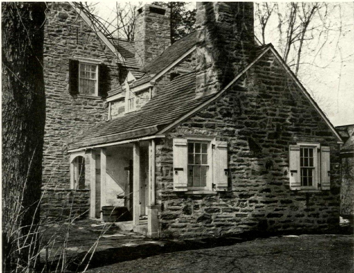
Detail from House of I. Wistar Morris, Esq., Chestnut Hill, Pa. Pennsylvania ledge stone with flush cement mortar pointing
