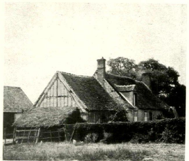
Old French Farmhouse at Anjou Showing small scaled tile roofs, stucco and half-timber walls
