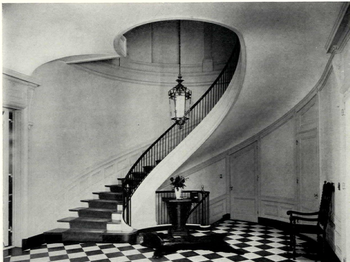
A formal treatment of a curved stairway with the iron railing set on a closed string
