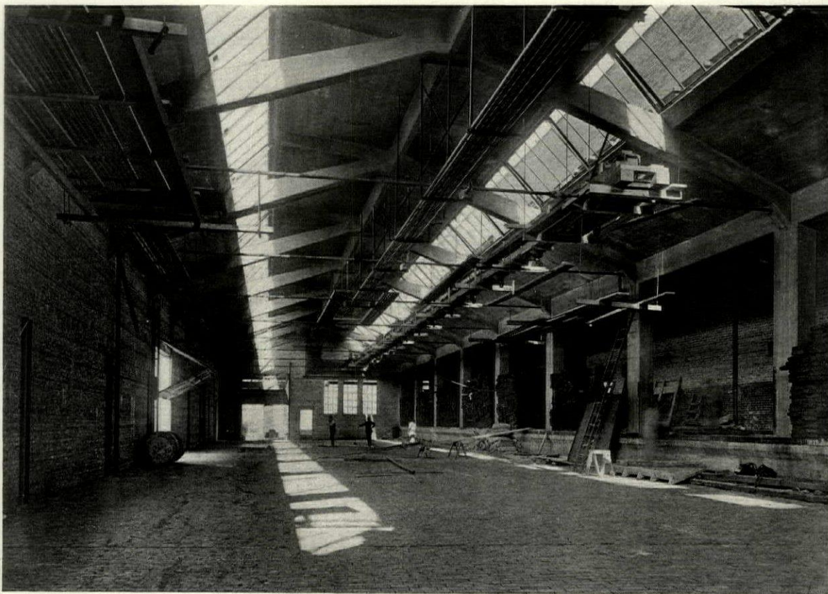
Combined Shipping Court and Garage, Hydrox Co. Ice Cream Factory, Chicago Electric trucks are used exclusively and connections for charging are provided overhead Richard E. Schmidt, Garden & Martin, Architects
