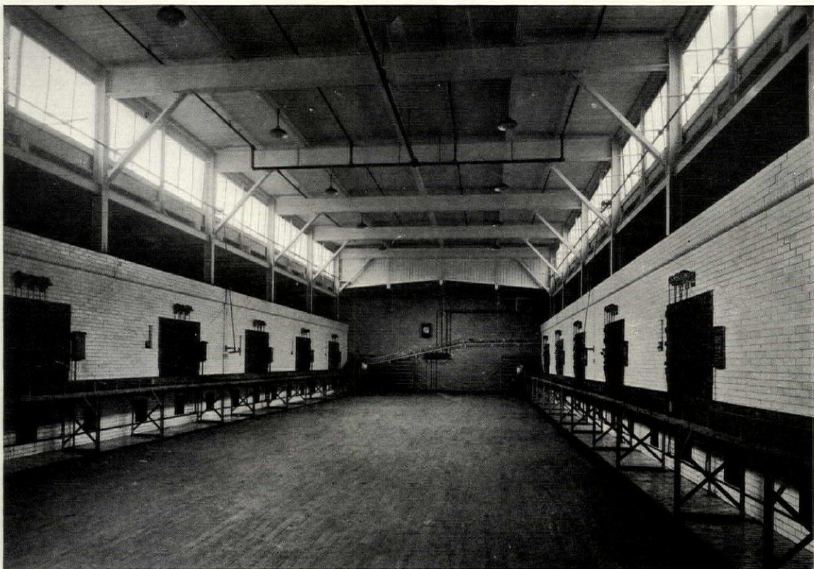
Baking Room, General Baking Co. Plant, Bronx, New York Simple monitor roof supported by steel beams. Note appliance for opening sash The Ballinger Company, Architects and Engineers
