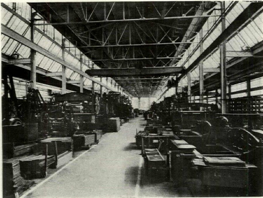
Interior of heavy stamping mill showing typical steel "mill building" construction with craneway under monitor. Plant of Edw. G. Budd Mfg. Co., Philadelphia The Ballinger Company, Architects and Engineers
