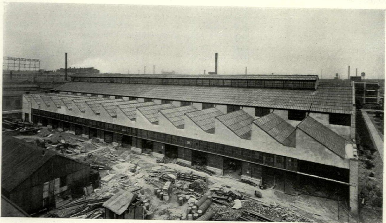
Maxwell Motor Company Plant, Detroit Saw-Tooth and Monitor Type Roofs Covered with Interlocking Cement Tile with Glass Insert Slabs
