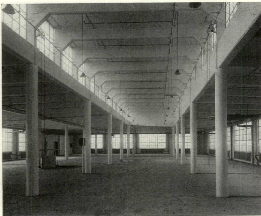
Concrete Monitor Construction with Movable Steel Sash Tiffin Building, Long Island City, N. Y. The Ballinger Company, Architects and Engineers
