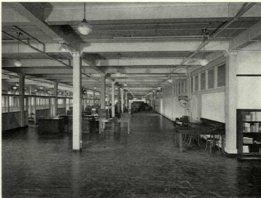
Interior of office section of The Chilton Company Building, Philadelphia, showing heavy mill construction, inexpensively finished
