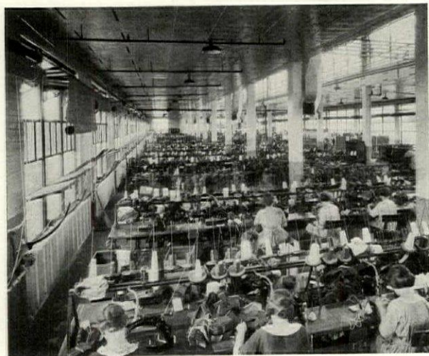
H. C. Goodman Shoe Factory, Columbus, O. Wall Radiation and Ventilation from Ducts in Monitor
