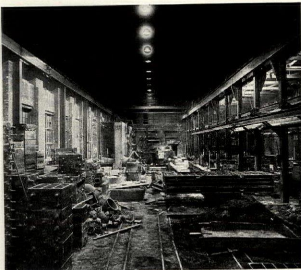
Fig. 5. Night view of a foundry lighted by 300-watt clear lamps in standard dome reflectors, 35 feet above floor; 10-foot centers in 40-foot bays. Resultant intensity is 5-foot candles
