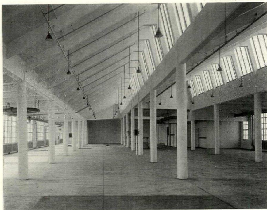
Concrete Saw-tooth Construction with Fixed Sash Tiffin Building, Long Island City, N. Y. The Ballinger Company, Architects and Engineers
