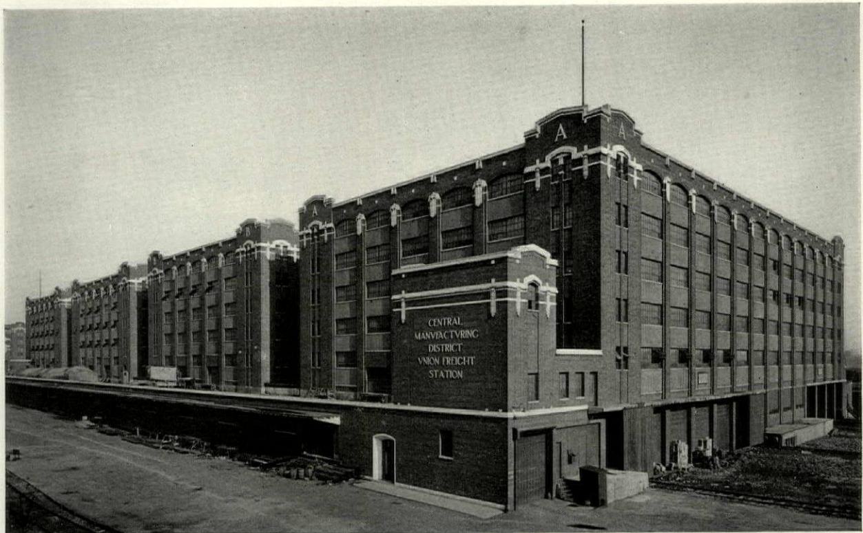
Group of four standardized warehouses with shipping facilities and railroad sidings in basement. Flat slab reinforced concrete construction. Central Manufacturing District, Chicago
