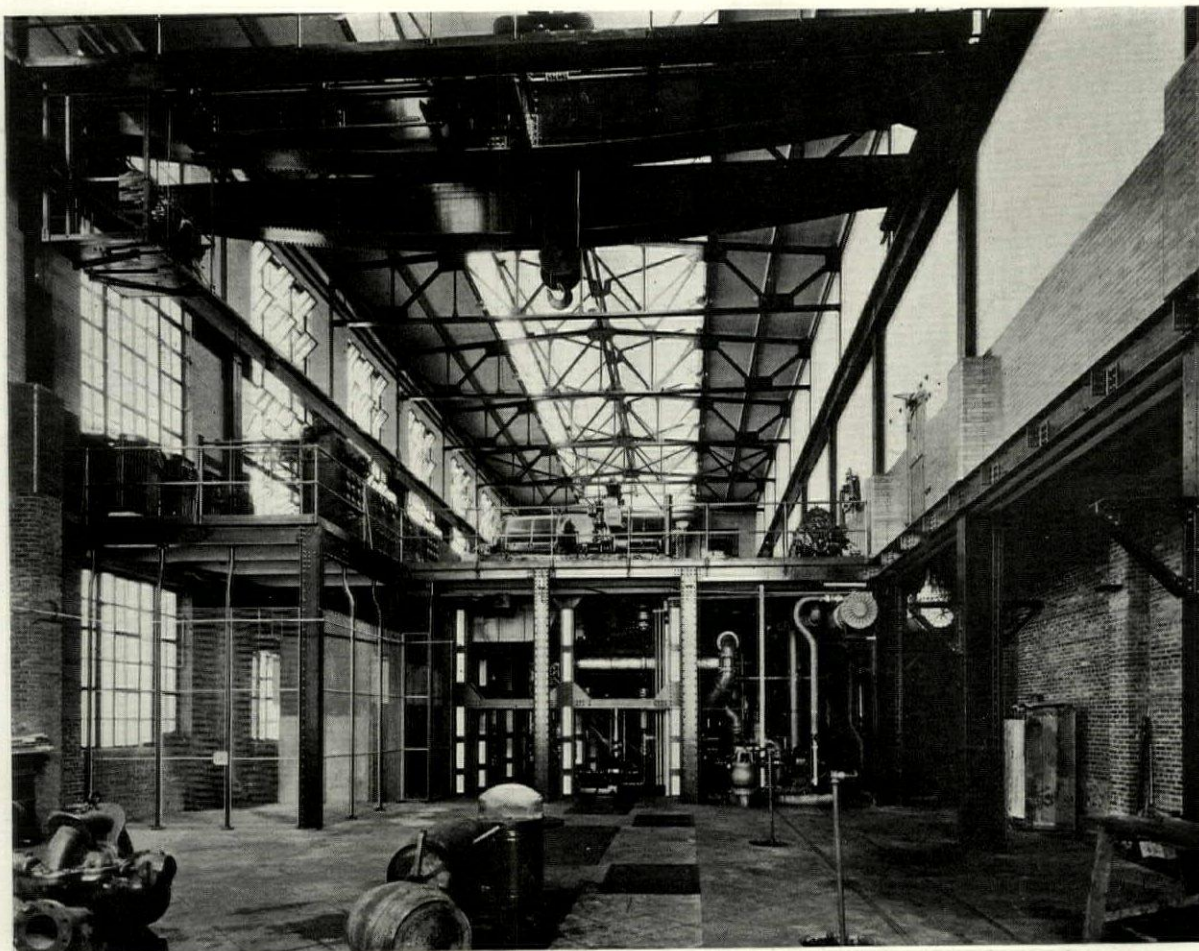
Interior of Power House, Victor Talking Machine Co., Camden, N. J. Crane extends across width of building with monitor above. The monitor roof drains to the center to assist conducting warm air and gases out through the ventilating sash The Ballinger Company, Architects and Engineers
