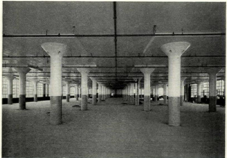
Interior of James Lees & Sons Co. Factory, Bridgeport, Pa., showing excellent light obtained from continuous sash; building 121 feet wide
