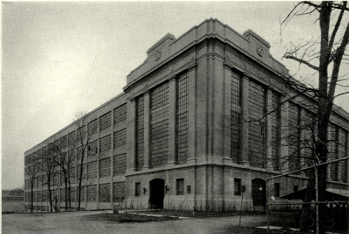
Detail of Corner Pylon, Siege Building, U. S. Arsenal, Rock Island, Ill. Reinforced concrete construction with architectural features of concrete cast in place. The main facade is 600 feet long
