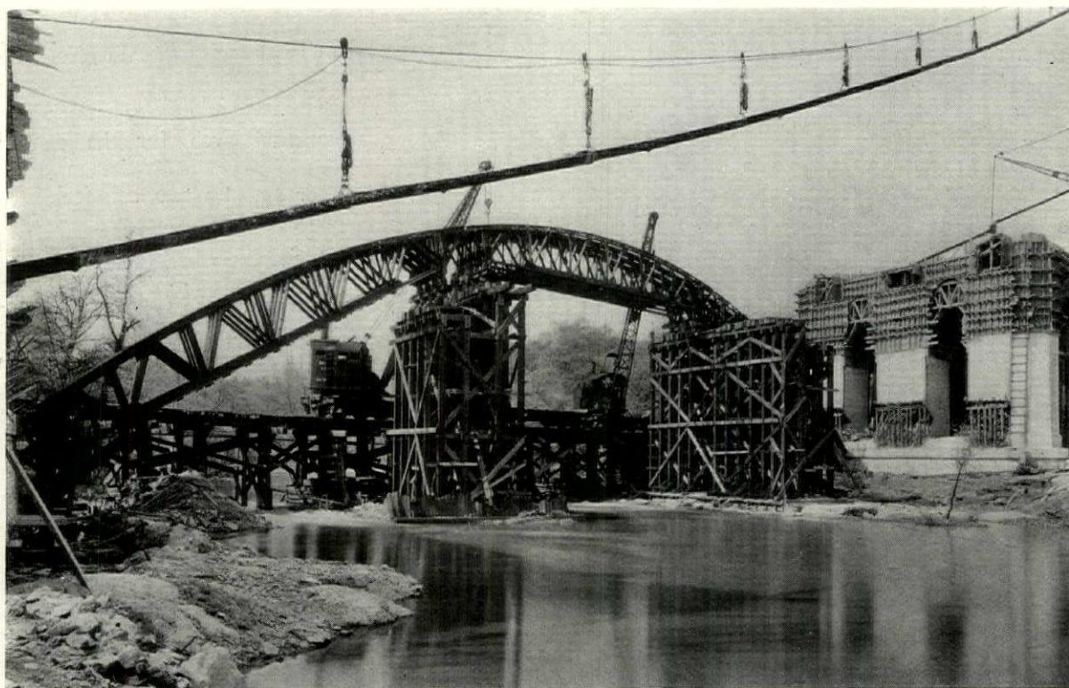
Steel Centering for Arch Ribs of Central Span
