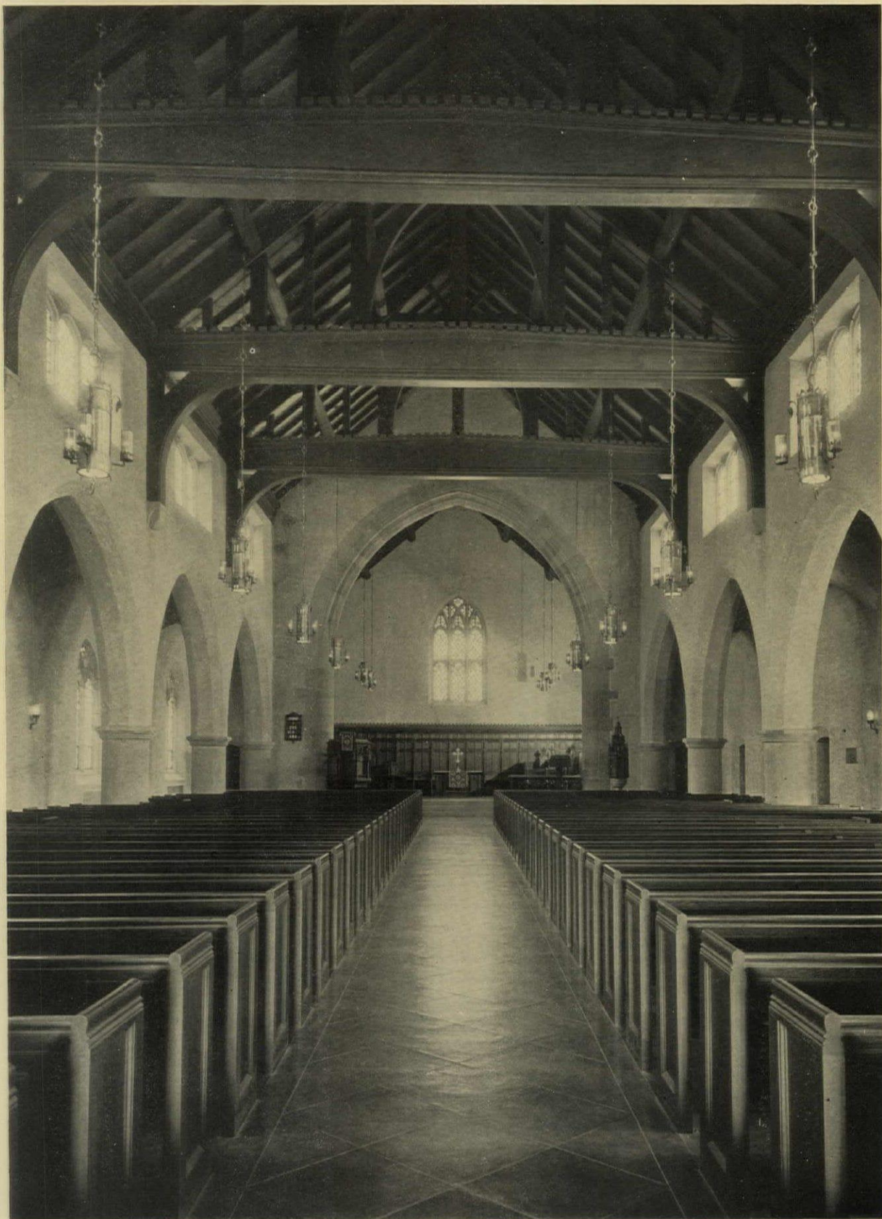
THE NAVE REFORMED CHURCH, BRONXVILLE, N. Y. HARRY LESLIE WALKER, ARCHITECT
