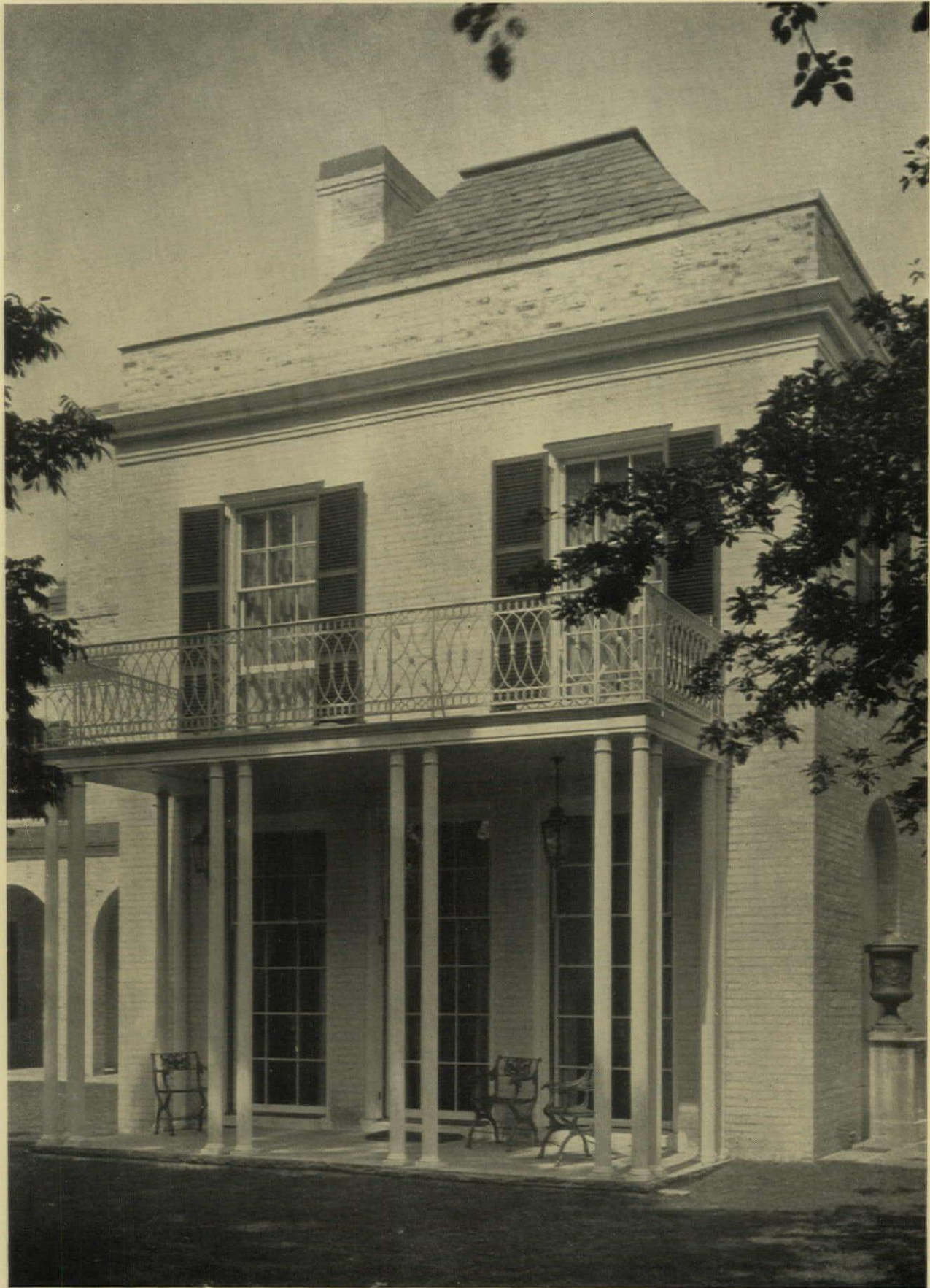
DETAIL OF SOUTH PORCH HOUSE AT PURCHASE, N. Y. LEIGH FRENCH, JR., ARCHITECT
