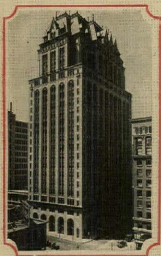
Coast Division Building, Pacific Telephone & Telegraph Co., San Francisco
