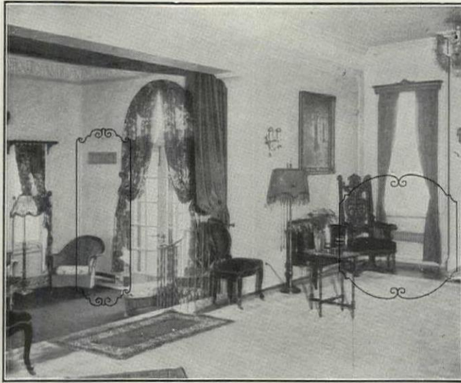
Living Room in the W. E. Hyde Residence, Memphis, Tennessee
