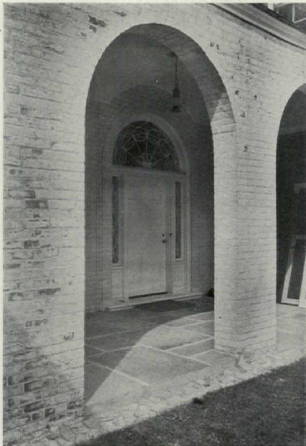
Main Entrance Door
