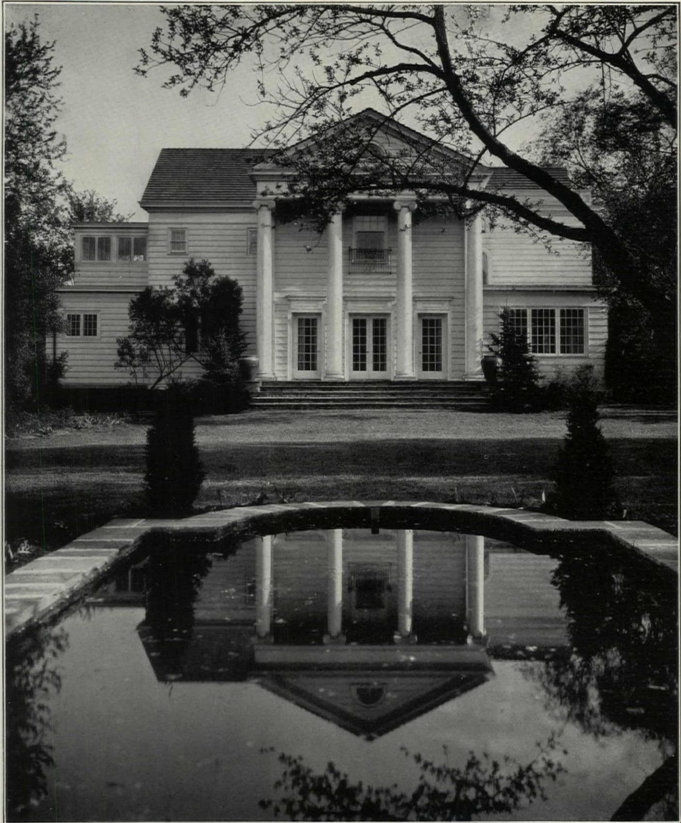
Residence of W. H. MALONE, Park Ridge, Ill. Zook and McCaughey, Architects
