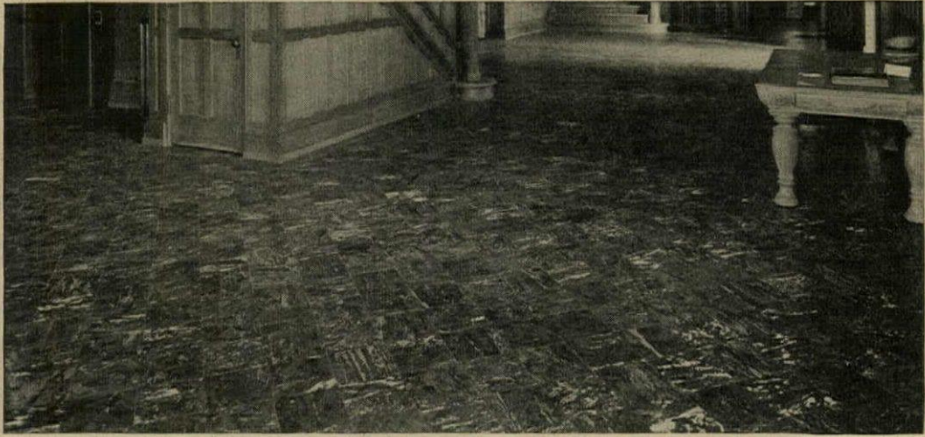
Effective use of Goodyear Rubber Tiling in basement of First Presbyterian Church at Buffalo, New York Installed by Griffiths Floor Company, Buffalo
