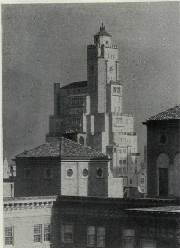
PARK LANE HOTEL (in Foreground) SCHULTZE & WEAVER, ARCHITECTS
