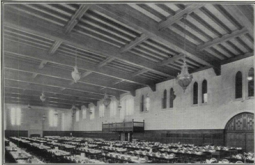
Dining Room, Notre Dame University, South Bend, Indiana. Here Acousti-Celotex tiles add to the permanency and beauty of the ceiling. Also, the tiles quiet all sounds resulting from the crashing of trays, rattle of dishes and clamor of conversation. Cram & Ferguson, architects; Arc-Con Specialties Company, Acousti-Celotex contractor.
