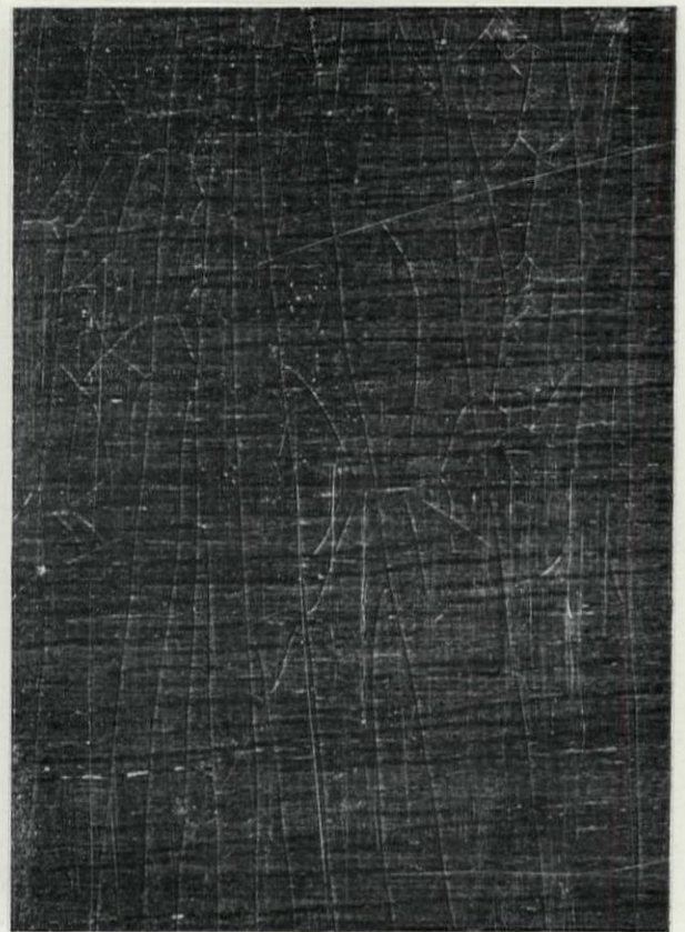
Old Age or "Crow-foot" Cracks
