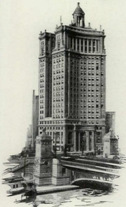
London Guarantee & Accident Co. Bldg., in Chicago, is one of the late prominent ATHEY-weatherstripped installations.
