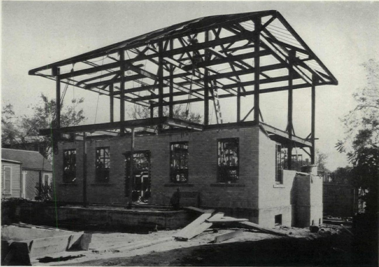
Steel Frame, House of Frank G. Clark, Baton Rouge, La.
