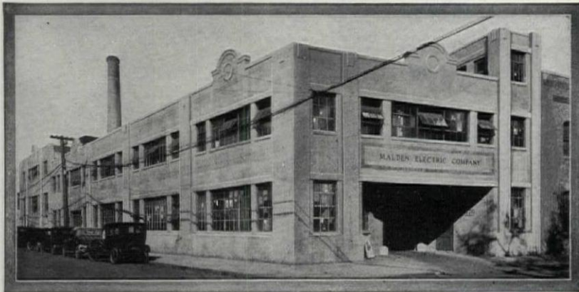
The 115 car Garage of the Malden Electric Company, Malden, Mass., erected to house their fleet of trucks and service cars.
