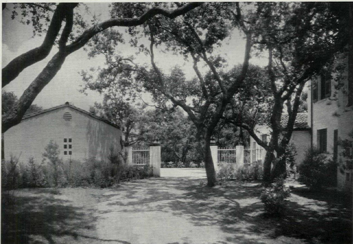
GARAGE AND GATEWAY TO SERVICE COURT HOUSE OF O. N. GABRIEL, ESQ., SAN MARINO, CALIF. ROLAND E. COATE, ARCHITECT
