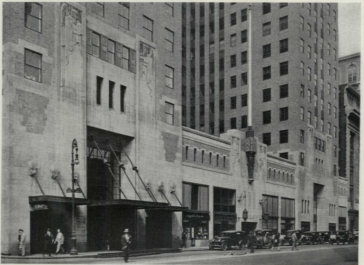
An Unusually Interesting Treatment Gives Variety and Decoration to the Lower Stories of the Graybar Building, New York
