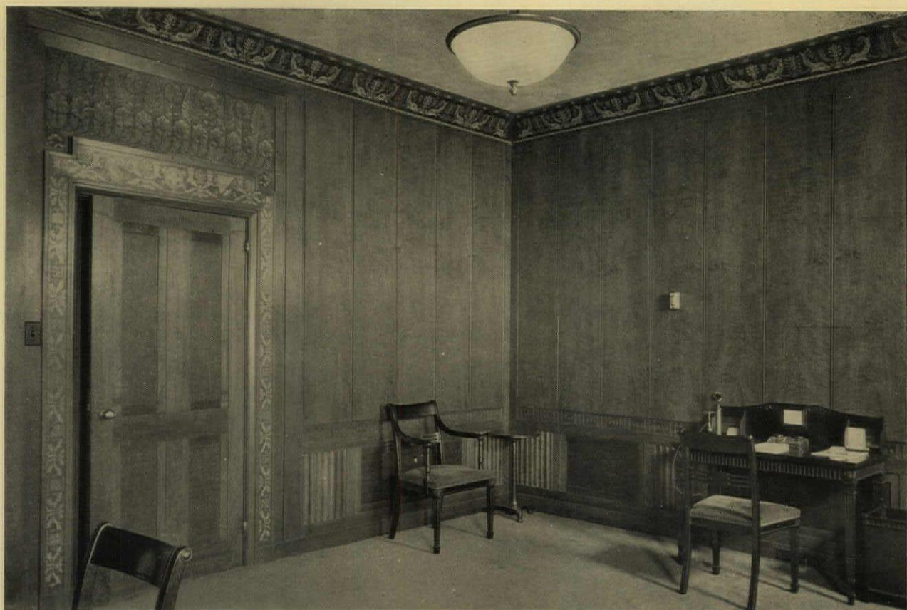
TELEPHONE ROOM, TWENTY-SIXTH FLOOR
