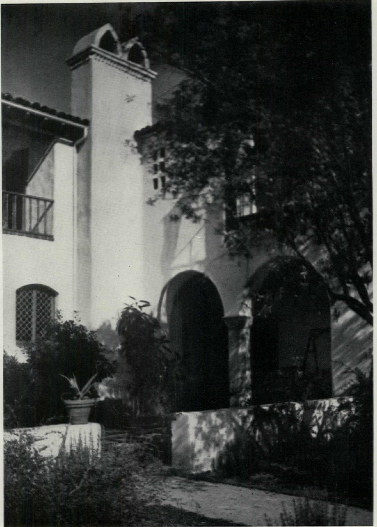
LOGGIA, HOUSE OF MILTON BARUCH, ESQ., HOLMBY HILLS, CALIF. - GORDON B. KAUFMANN, ARCHITECT
