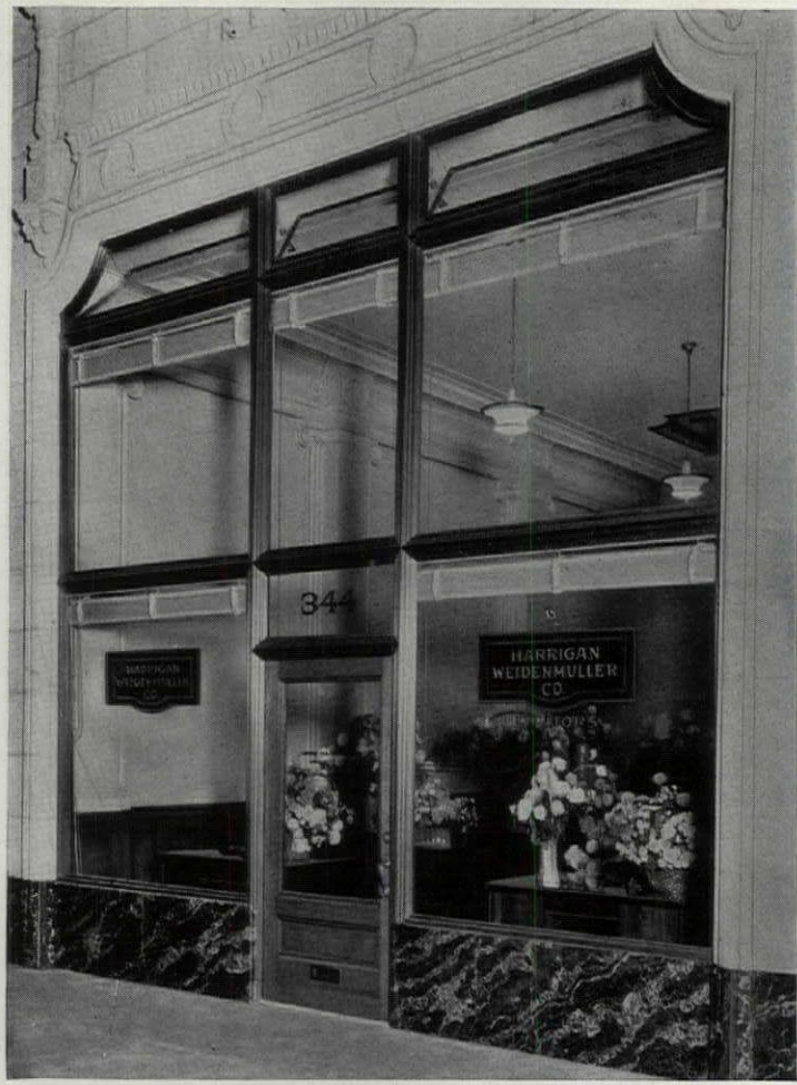
FREDERICK H. MEYER, Architect —K. E. PARKER CO., General Contractor SAN FRANCISCO
