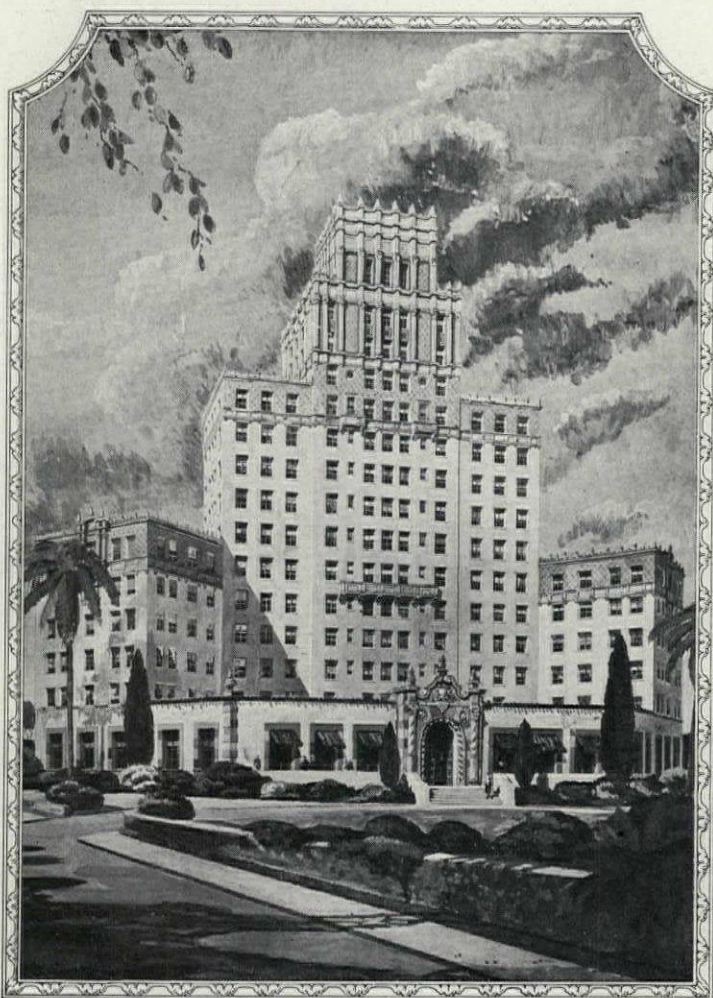
Walker & Eisen, Architects.
