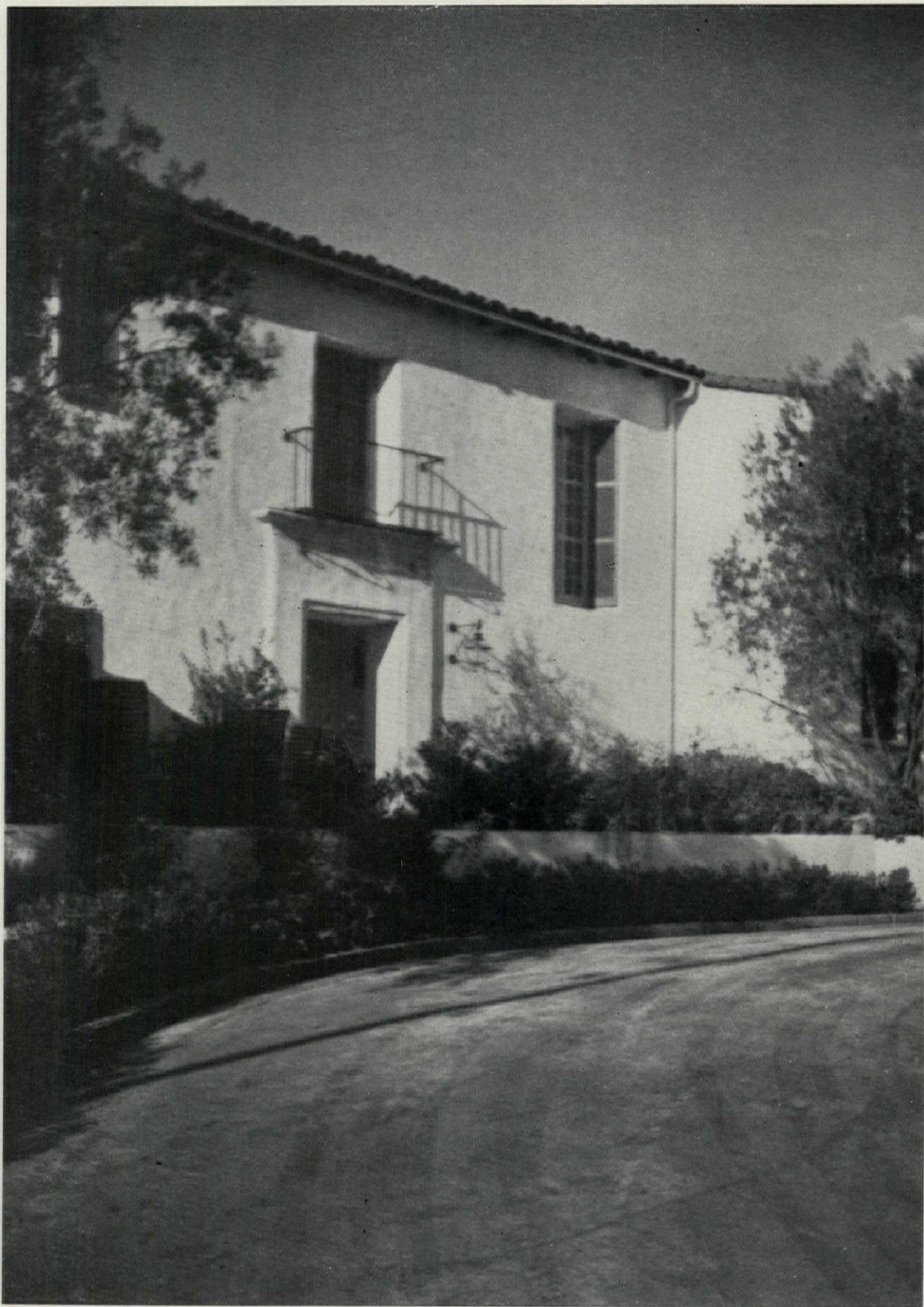
ENTRANCE, HOUSE OF MILTON BARUCH, ESQ., HOLMBY HILLS, CALIF. GORDON B. KAUFMANN, ARCHITECT
