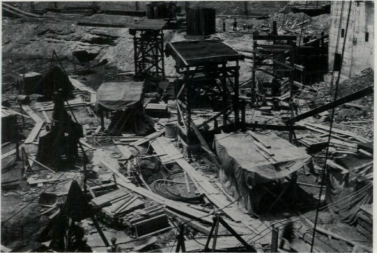
Square and Tripod Head Frames Over Many Wells for the Foundations
