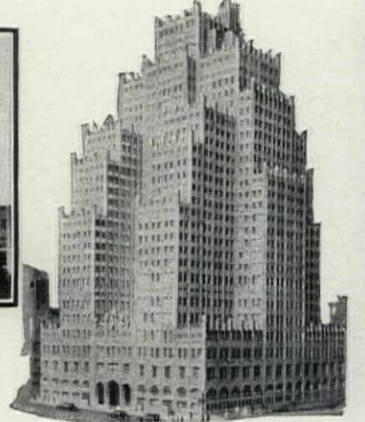
ST. LOUIS Bell Telephone Building
