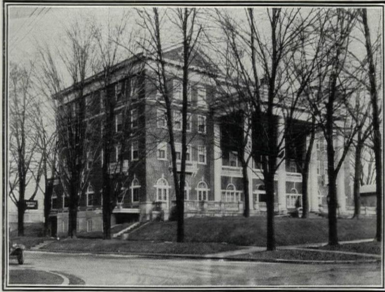
New Parker Inn, Albion, Michigan, equipped with McCRAY refrigerators
