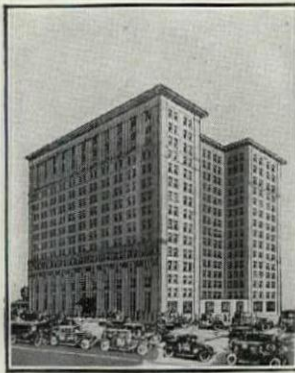
NEW ORLEANS Whitney Central Building
