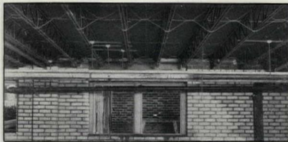
A close-up of a finished Havemeyer Truss floor. Pipes and conduits can be carried through the open webs of the trusses.
