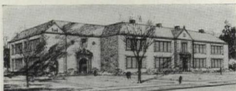
Independence School General Contractor—Wm. Donnelly Co.
