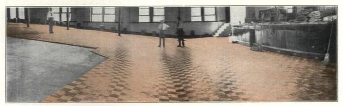
Each block is a complete unit, three or more oak strips, splined together. Each block is BruCELLized, a marvelous chemical process developed in the Bruce laboratories, which prevents shrinking or swelling, and increases durability. As a result, the floor will remain firm and level, and as the mastic is sound-deadening, is more quiet than any other permanent floor covering. Low cost, lowest maintenance, together with distinctive beauty, are now possible in school floors for rooms of any area.
