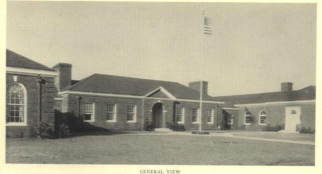
The simplicity of the Colonial design used here is very pleasing in a school of this type. Being all on one floor and designed for a capacity of 385 students, it necessarily covers considerable area and is laid out with two wings containing classrooms on either side of the central section in which are located the library, assembly room, teachers' and principal's rooms and some classrooms.
