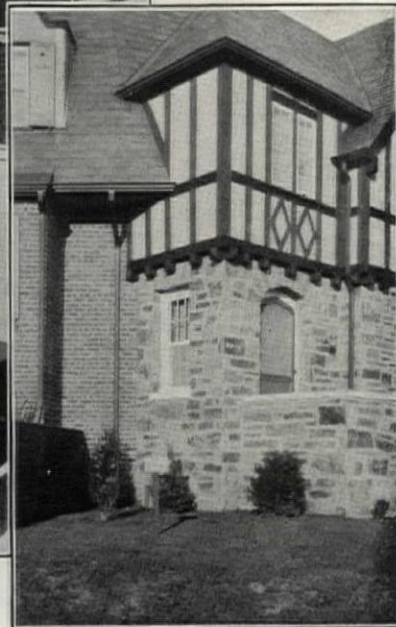
Exterior of a house in Foxhall Village. Cinder Blocks have been used as a base for stucco and as backing for stone and brick work, as well as for all partition walls.
