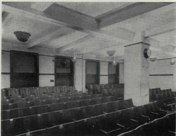
Totally Indirect Lighting Provides 10-Foot Candles at Chair-tops
