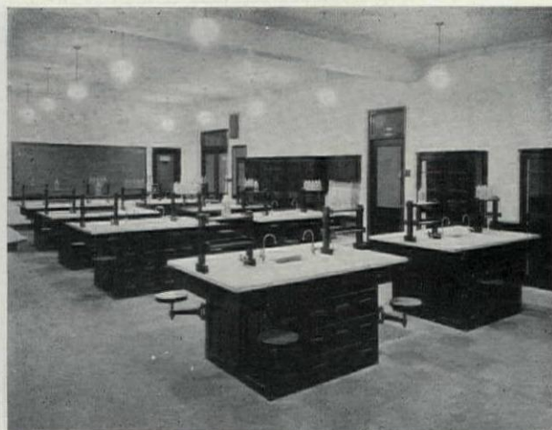
Prismatic Glass Direct Lighting Luminaries; Illumination 10-Foot Candles Schenck & Williams, Architects
